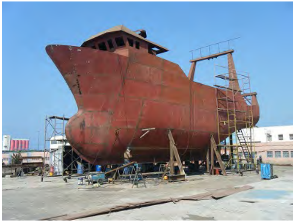
Fishing Vessel under construction at Shipyard
