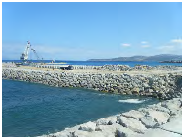
Fishing Port, under Construction,
