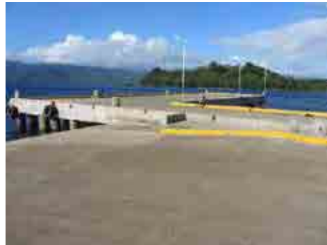
Figure 4-29 Newly constructed mooring jetty at SavuSavu Jetty
