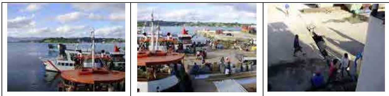
Figure 4-57 Internal quay of Port of Port-Vila (Star Wharf)
