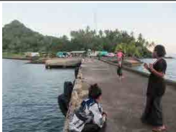
Figure 4-22 Natovi Jetty before arrival of a ferry
