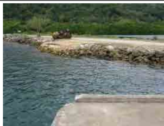
Figure 4-59 Approach road and ramp of Lits Lits Wharf
