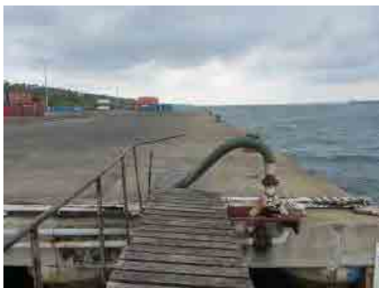
Figure 4-64 New quay of the Main Wharf of Port of Luganville
