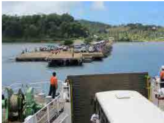
Figure 4-26 Entire view of Nabouwalu Jetty
