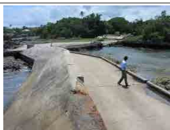
Figure 4-63 Approach road to Lenakel Wharf
