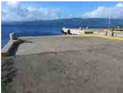
Figure 4-28 Ramp of SavuSavu Jetty to which Ro-Ro boats are moored (longitudinal mooring)
