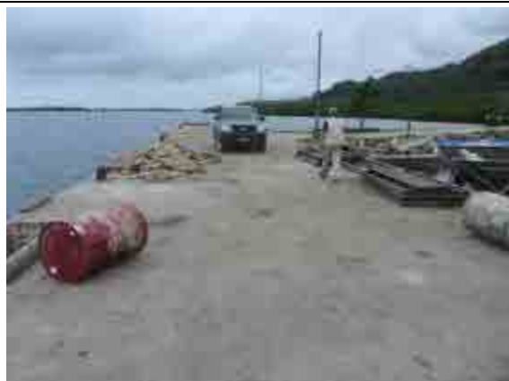
Figure 4-58 Entire view of Lits Lits Wharf (T-shaped pier)
