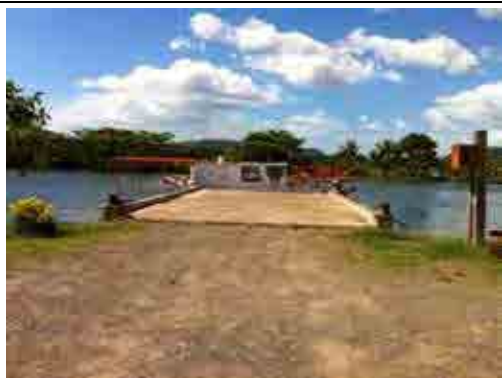
Figure 4-30 Entire view of Labasa Jetty
