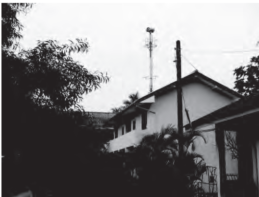
Tsunami EW Tower Location
