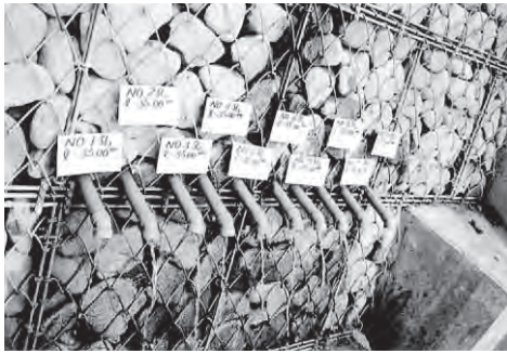
Figure 3.4.5 Horizontal drainage work
