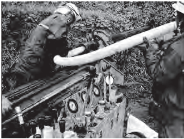
Figure 5.6.2 Flushing of Drainage Pipe
