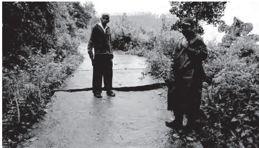
Figure 4.2.1 Appearance of new crack at Mahawewa
