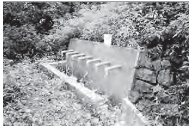
Figure 5.3.6 Outlet of Horizontal Drilling
