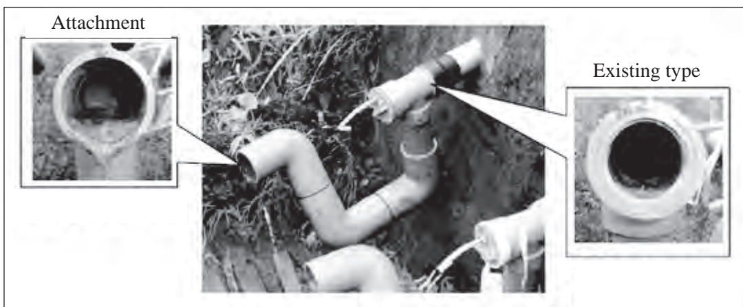
Figure 5.6.3 Pipe Outlets which prevent Water Clogging
