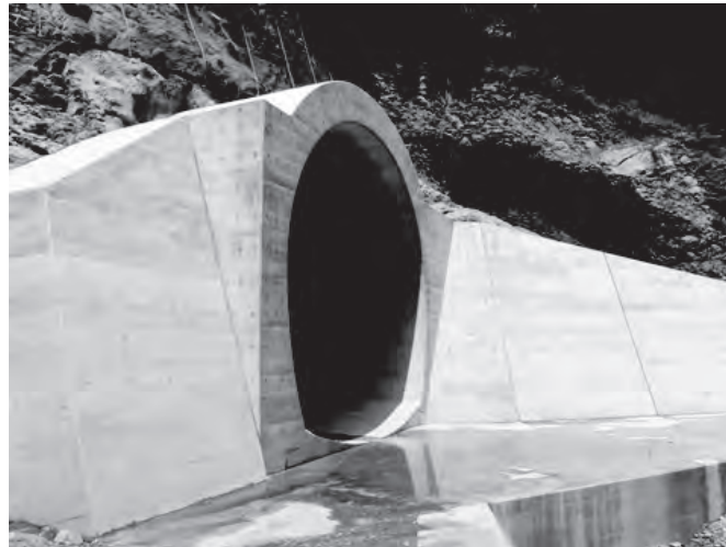
Figure 3.4.10 Drainage tunnel work *4
