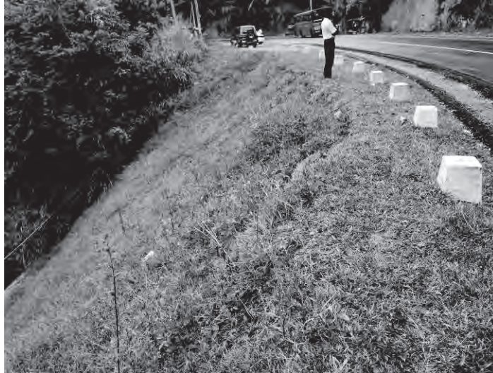
Figure 4.2.2 Heaving of Embankment at Permadulla
