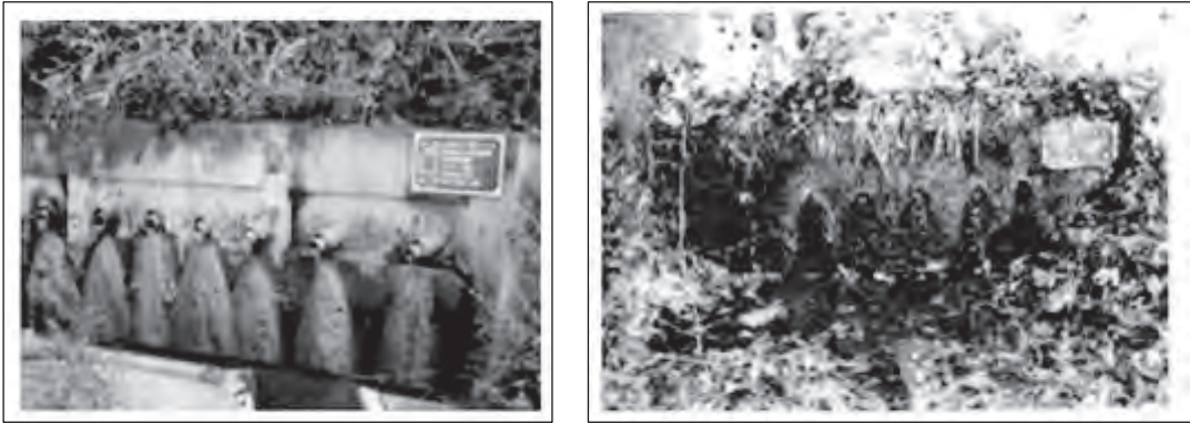
Figure 5.6.1 Clogged Drainage Pipes
