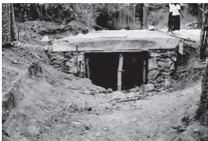
Photo 33 Installation of Small Water Drainage at the Community (Matale)
