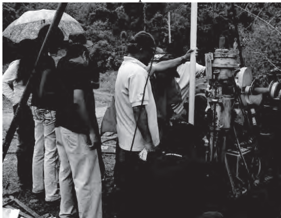
Photo 19 Installation of Monitoring Equipments
