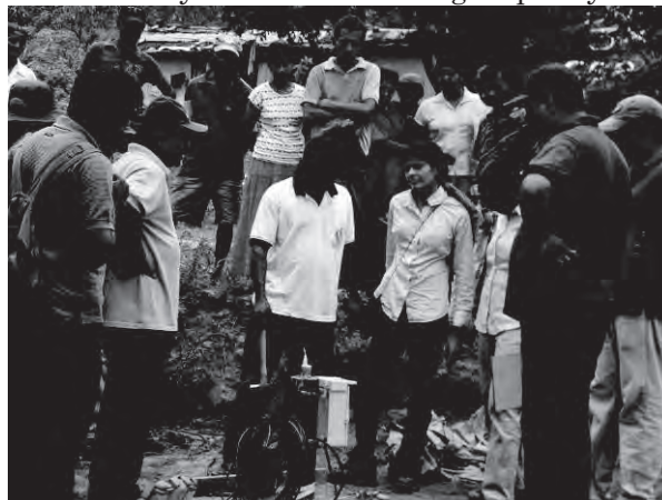
Photo 20 Installation of Monitoring Equipments
