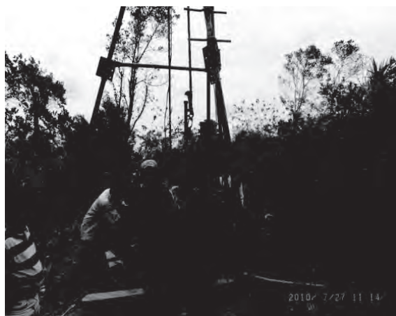
Photo 21 Installation of Monitoring Equipments
