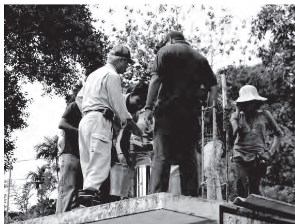
Photo 22 Installation of Monitoring Equipments
