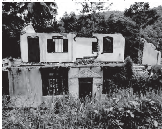
Photo 8 Site Survey in the flood affected area
