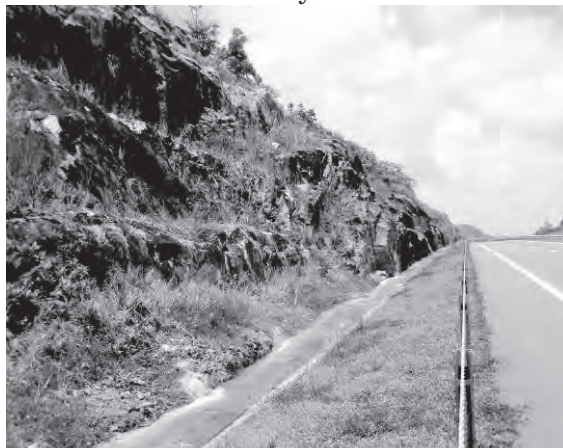
Photo 2 Disaster Site Visit on DIA
