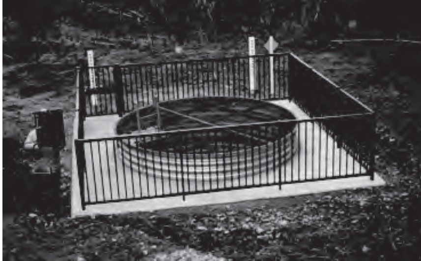
Figure 3.4.9 View of a drainage well at the surface *5
