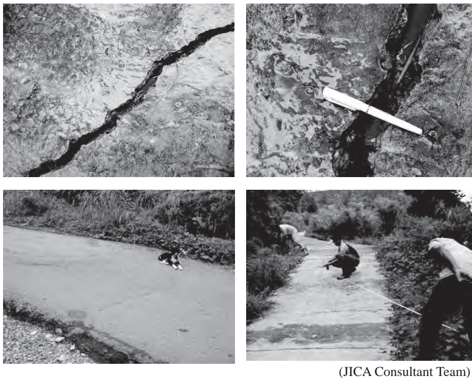
Figure 2.4.20 Measuring the distance between cracks
