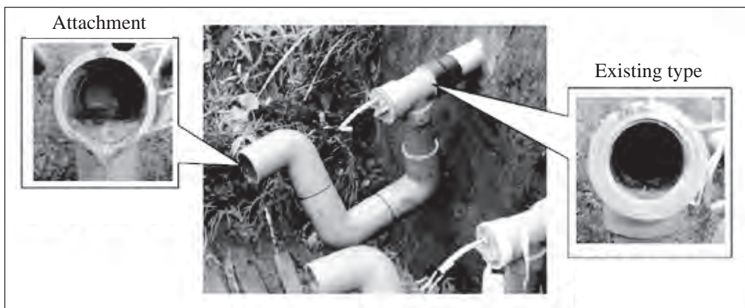
Figure 5.6.3 Pipe Outlets which prevent Water Clogging
