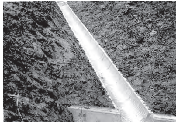
Figure 3.4.2 Corrugate water path
