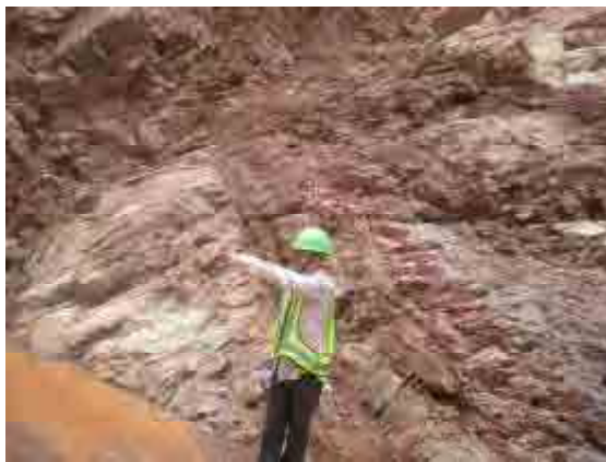
Checking the rock condition at Nam Luok Dam
