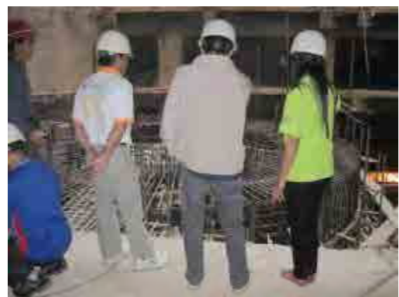
Site inspection for powerhouse
