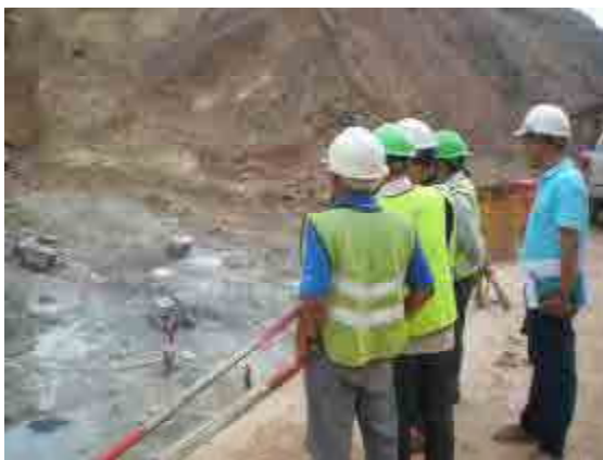
Grouting works at Nam Ken Dam
