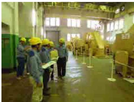
OJT at hydropower station
