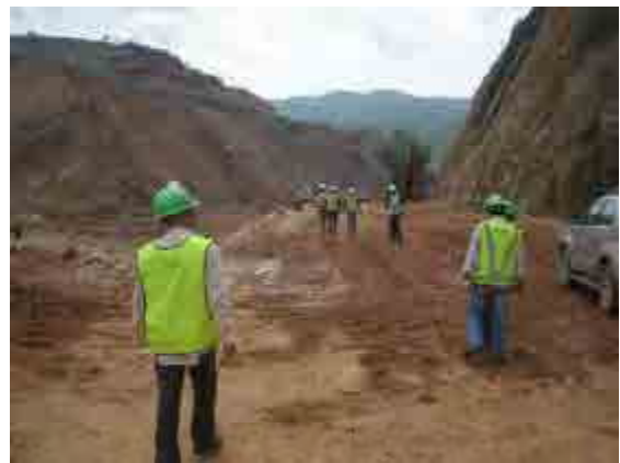
Site inspection at Nam Ken Dam
