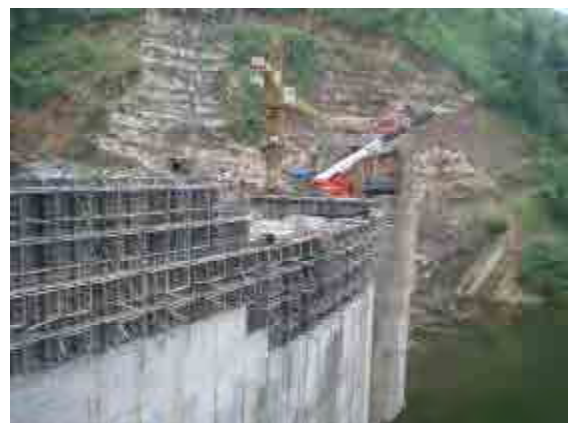
Installing spillway gates
