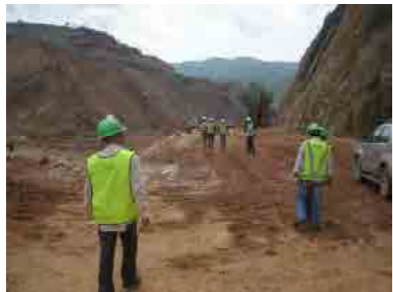
Site inspection at Nam Ken Dam
