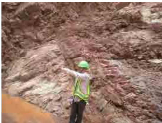
Checking the rock condition at Nam Luok Dam
