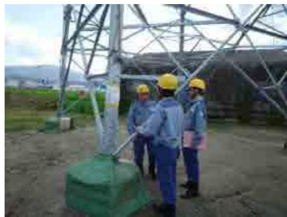
OJT (Sakurai line construction site)
