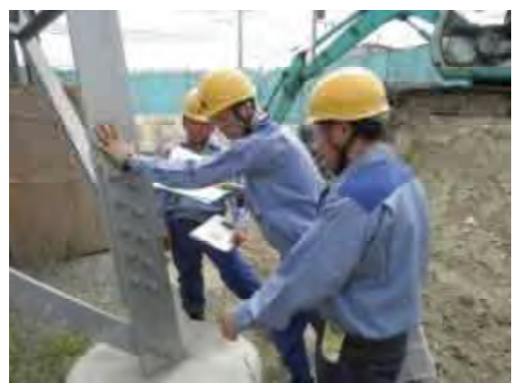
OJT at TL construction site
