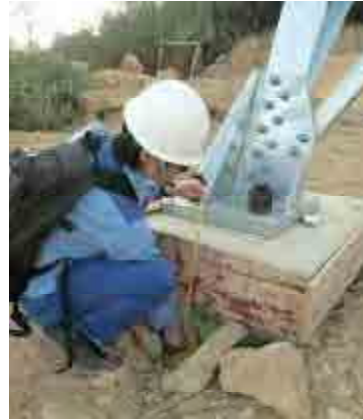
Site inspection for transmission line
