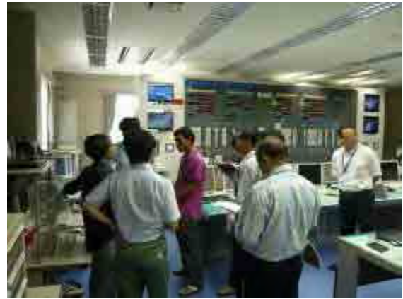
OJT at Koshido Dam Control Office
