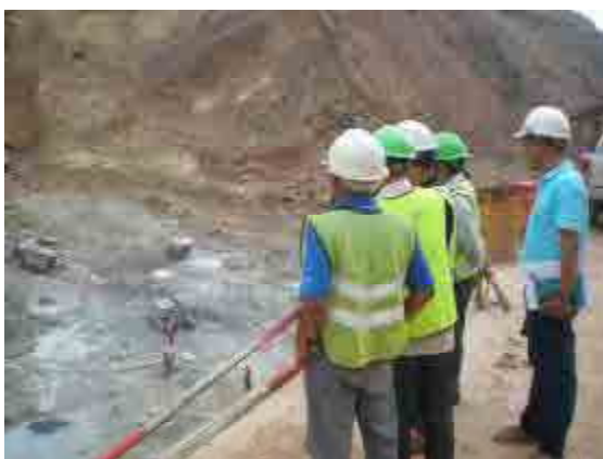
Grouting works at Nam Ken Dam
