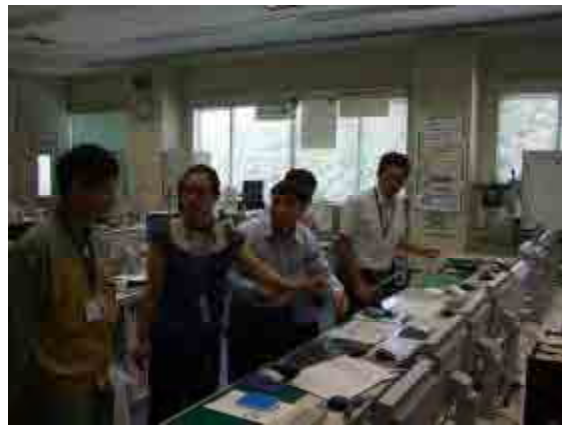
OJT at Koshido Dam Control office
