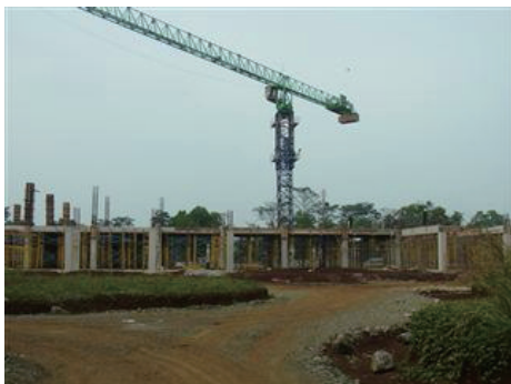
MCCOE construction site
