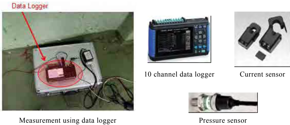
Figure 5- 42 Measurement of Operation Conditions of Air Compressor using Data Logger
