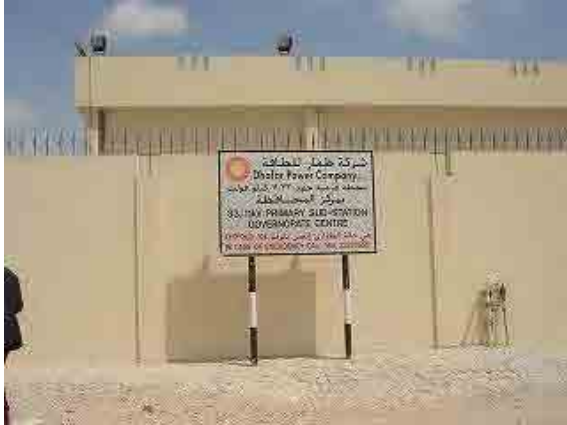
(a) Aspect of Primary Substation
