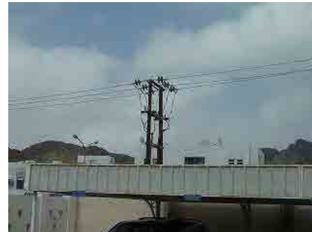
Figure 4- 13 11 kV Overhead Lines (MEDC)
