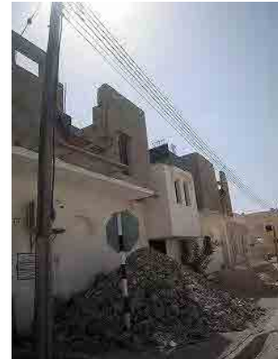
Figure 4- 14 Overhead Low Voltage Lines (DPC)
