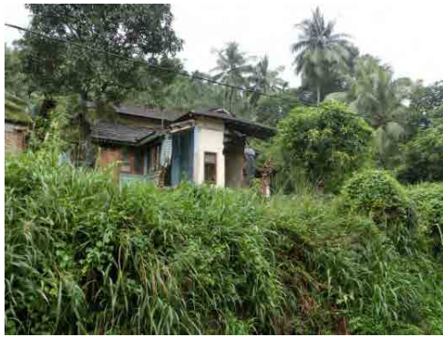
Photo-9 Half Collapse House by Landslide
