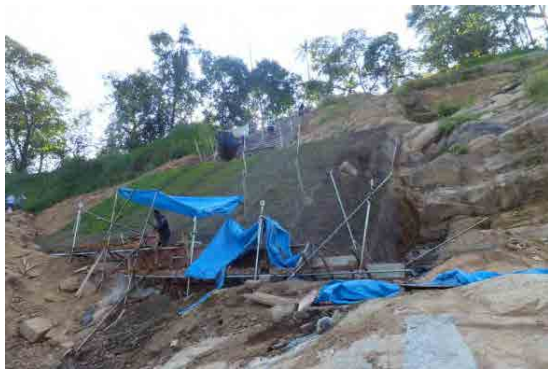
Photo-7 Situation of Countermeasure Construction
