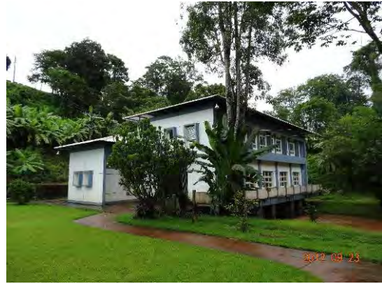
(9) O'Chum No.2 Power Plant Building: Can generate only 820kW despite its nameplate output of 960kW due to deteriorated equipment.
