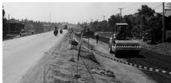
Pic.1 National Road No.1 Improvement Project
