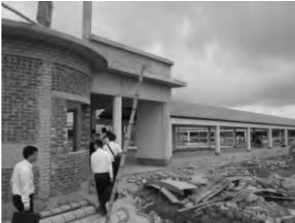
School under construction
