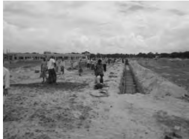
PAPs work for construction
