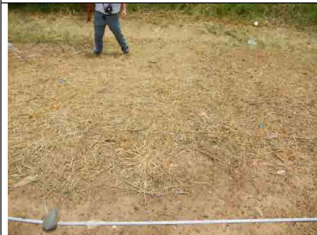
Photo-17: Sec. 7-1, 2 Gully erosion of Top Soil
