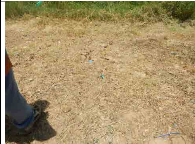
Photo-63: Sec. 20-4 Gully erosion of Top Soil and Dragon Hole
