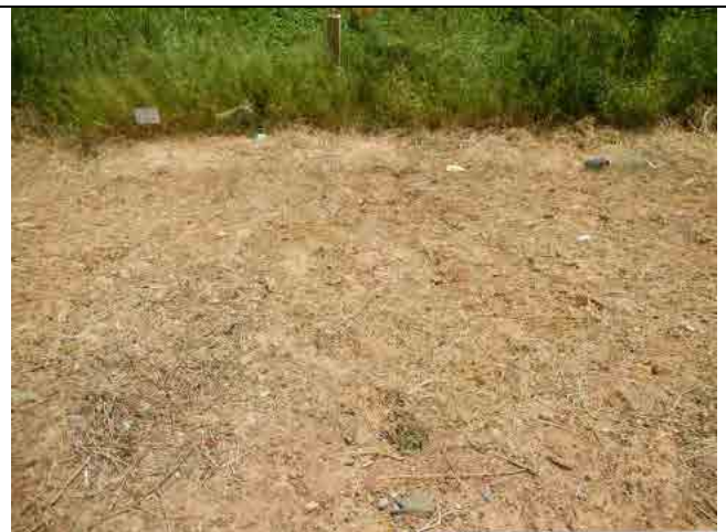
Photo-6: Sec. 3-1, 2, 3, 4 Gully erosion of Top Soil
