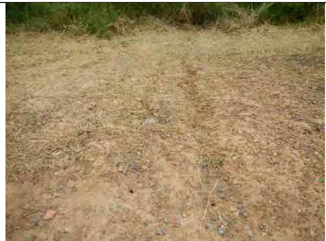
Photo-26: Sec. 10-1, 2 Gully erosion of Top Soil
