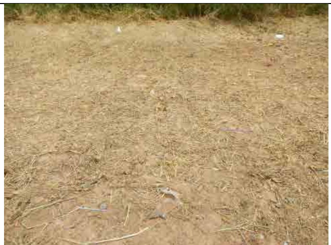
Photo-16: Sec. 6-4 Gully erosion of Top Soil
