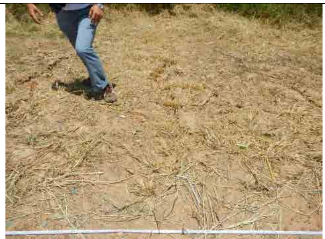
Photo-40: Sec. 14-2 Gully erosion of Top Soil
