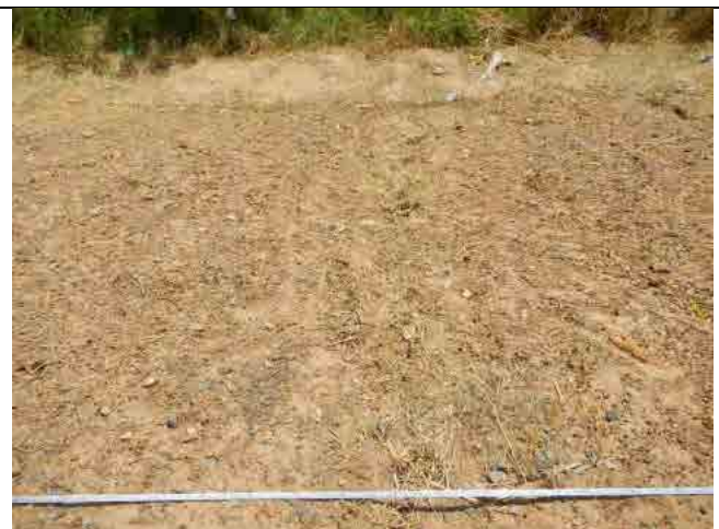
Photo-10: Sec. 4-4 Gully erosion of Top Soil
