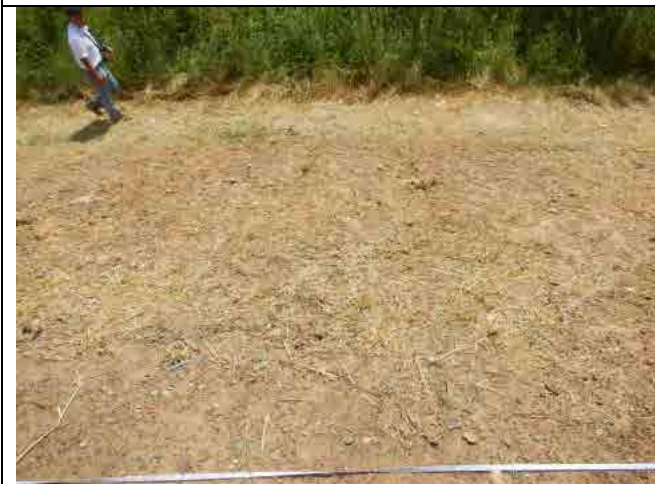
Photo-11: Sec. 5-1, 2 Gully erosion of Top Soil
