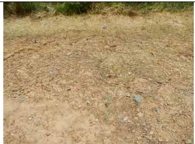
Photo-24: Sec. 9-3 Gully erosion of Top Soil
