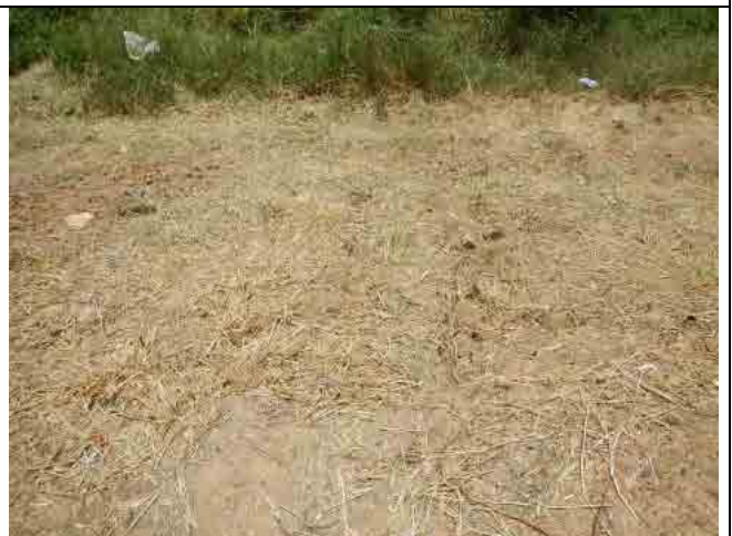
Photo-60: Sec. 19-5, 6, 7 Gully erosion of Top Soil
