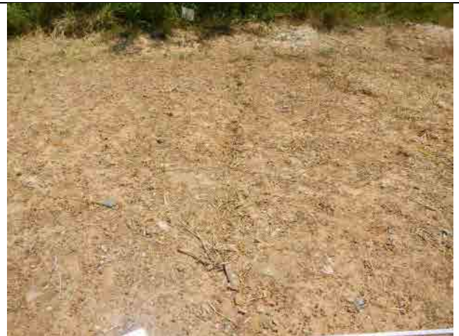
Photo-4: Sec. 2-2 Gully erosion of Top Soil
