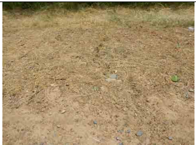
Photo-18: Sec. 7-3 Gully erosion of Top Soil
