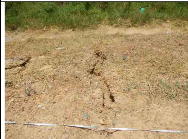
Photo-65: Sec. 21-2 Gully erosion of Top Soil
