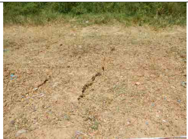
Photo-70: Sec. 23-1 Gully erosion of Top Soil
