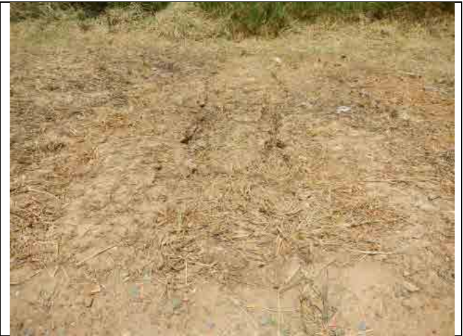
Photo-62: Sec. 20-2, 3 Gully erosion of Top Soil
