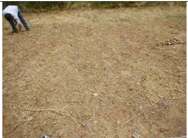
Photo-14: Sec. 6-1 Gully erosion of Top Soil
