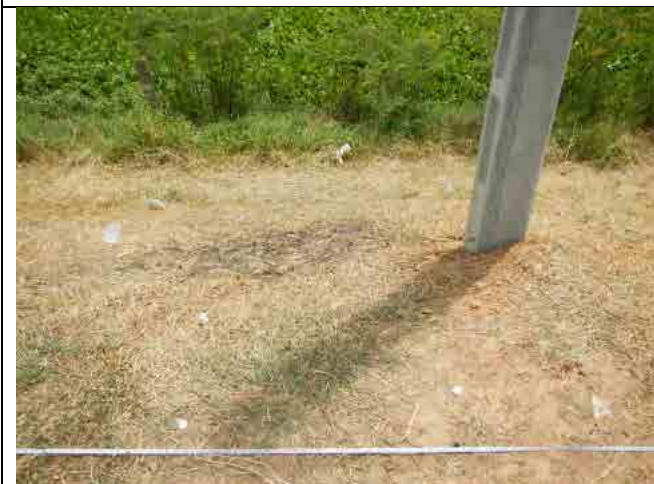
Photo-27: Sec. 10-3~5 Gully erosion of Top Soil
