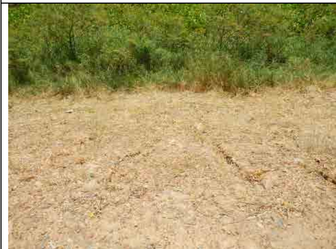
Photo-53: Sec. 18-3, 4 Gully erosion of Top Soil
