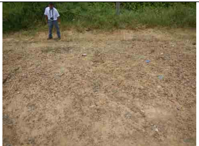
Photo-48: Sec. 17-1 Gully erosion of Top Soil
