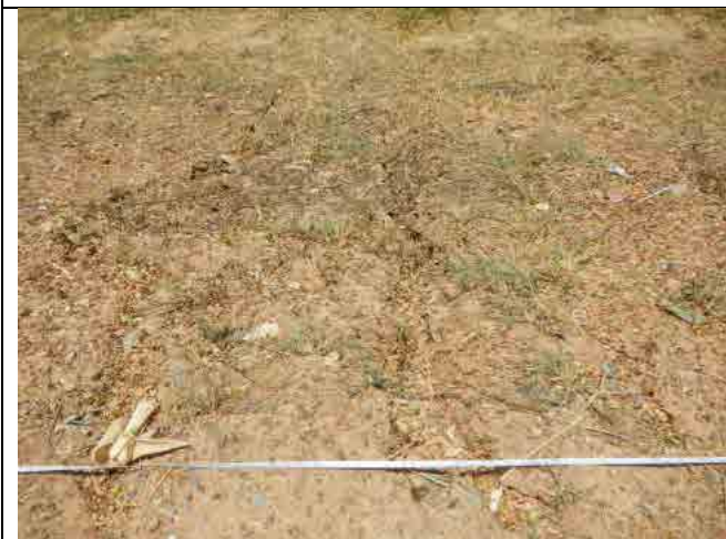
Photo-69: Sec. 22-5 Gully erosion of Top Soil
