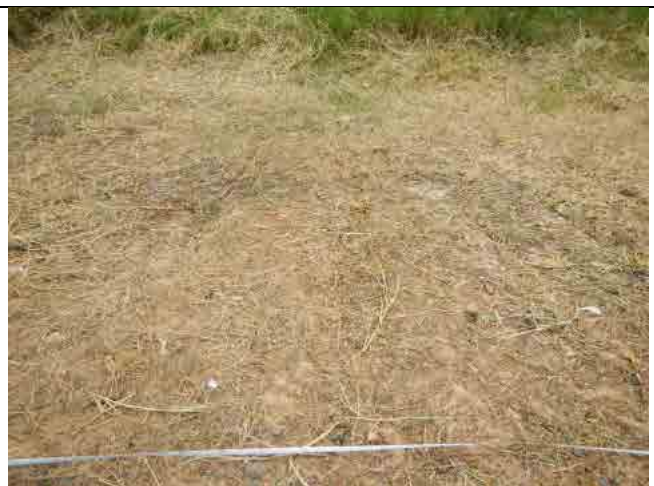
Photo-34: Sec. 12-3 Gully erosion of Top Soil
