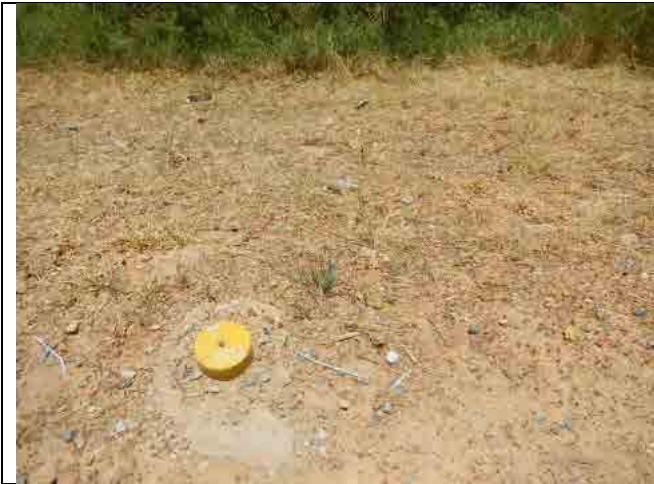
Photo-55: Sec. 18-6 Gully erosion of Top Soil
