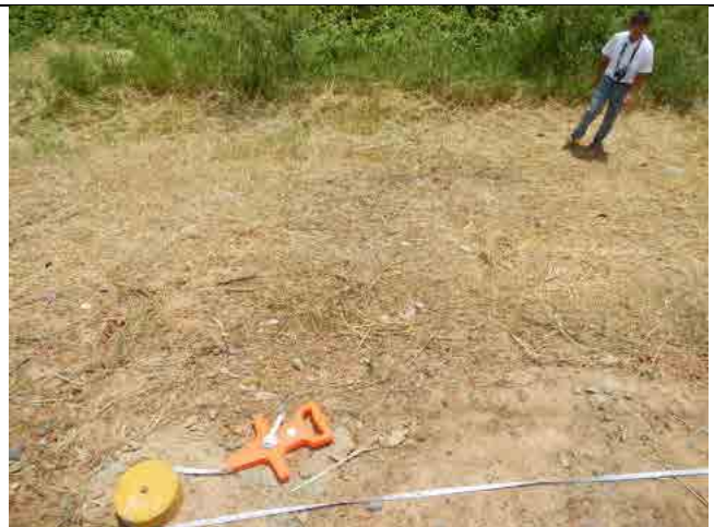
Photo-32: Sec. 11-4, 12-1 Gully erosion of Top Soil
