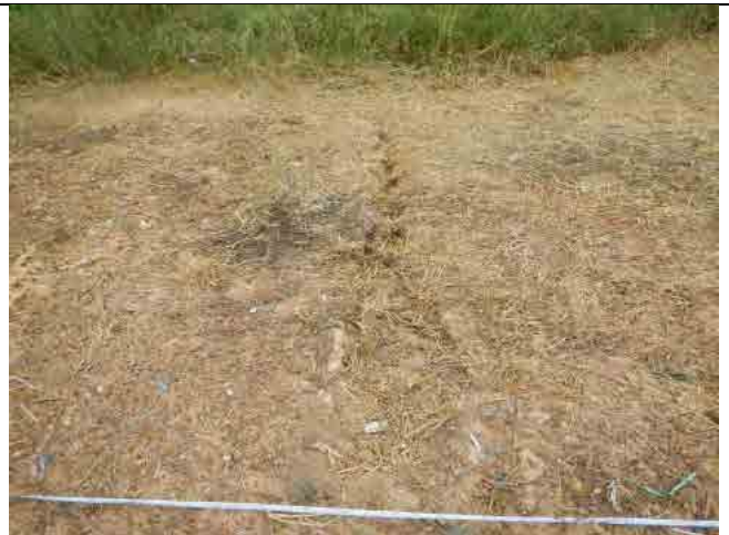
Photo-46: Sec. 16-2 Gully erosion of Top Soil
