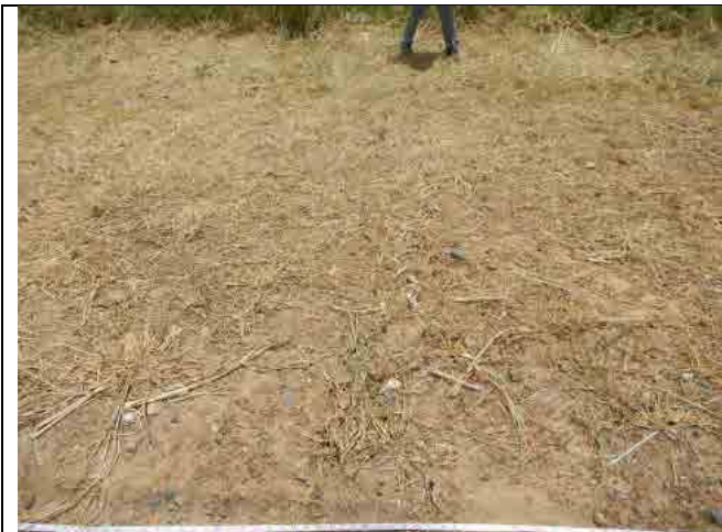
Photo-31: Sec. 11-3 Gully erosion of Top Soil
