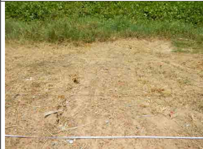
Photo-45: Sec. 15-4, 16-1 Gully erosion of Top Soil
