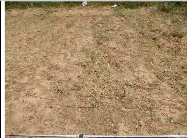
Photo-1: Sec. 1-1 Gully erosion of Top Soil
