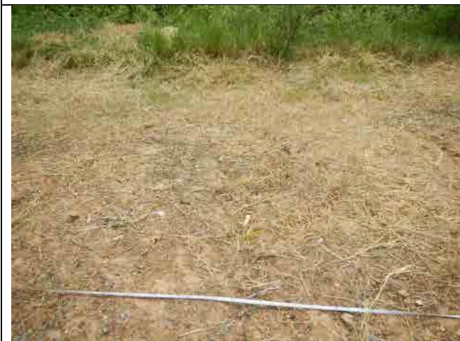
Photo-33: Sec. 12-2 Gully erosion of Top Soil
