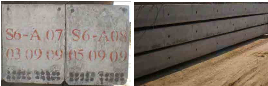
Precast PC Flat Slab Bridge
