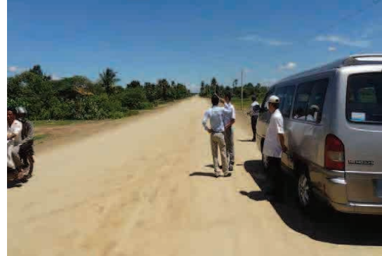
Completed Embankment at Termination
