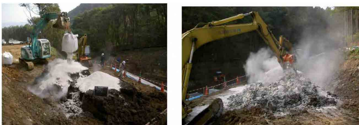
Photo 3.3-1 Mixing Soil with Additive
