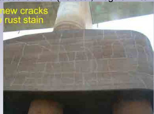
4.Observation (Cracks in P13) Multi-Column Foundation Footing (North Side) Latticed Cracks (Vertical, Regular Interval)
