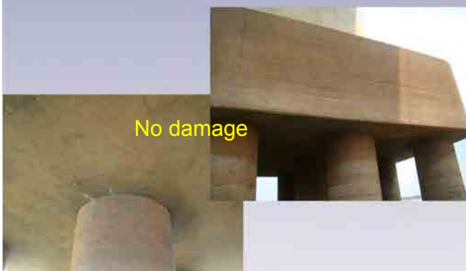
4.Observation (Other Footings)
