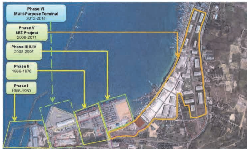
Source: Overview on Transport Infrastructure Sectors in Cambodia 2012
