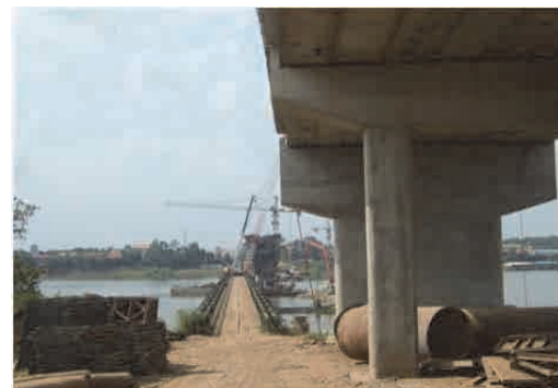
Photo of Bridge Construction
