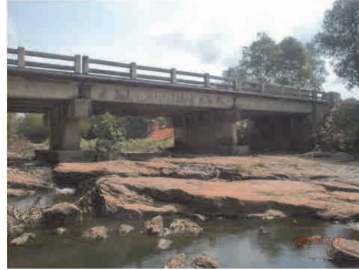
Bridge at PK 152.9
