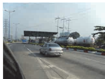
Photo (1) Toll Gate
