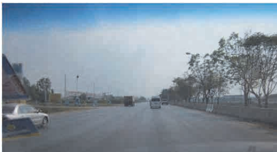
Lighting Post & Concrete Barrier
