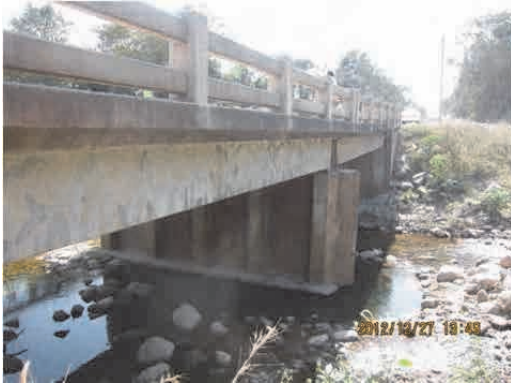
Bridge at PK 110.1
