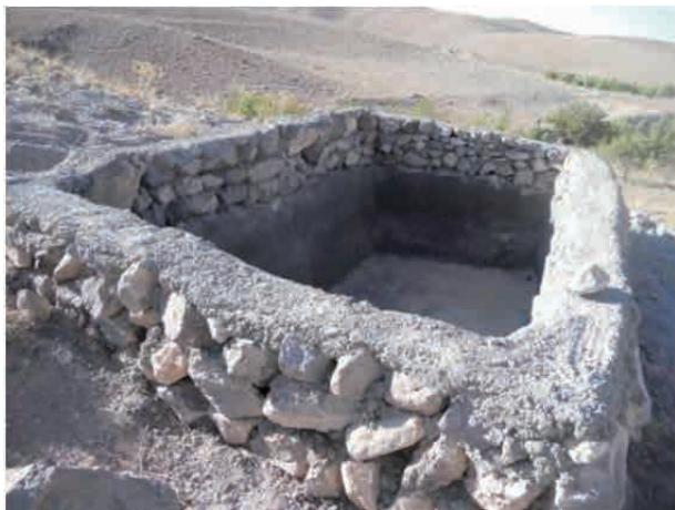
Water tank installed by the owner of the field ( V=7\sim 8\text{m}^3 )
