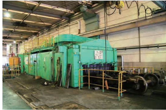
Source: JICA Study Team Figure 3.5.9 Bogie cleaning machine
