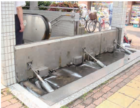
Figure 3.4.35 Example of water sealing plates
