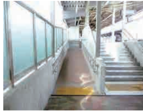
Source: JICA Study Team Figure 3.4.30 Handrail
