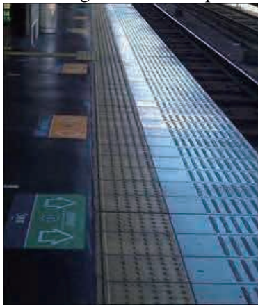
Source: JICA Study Team Figure 3.4.31 Braille blocks on the platform
