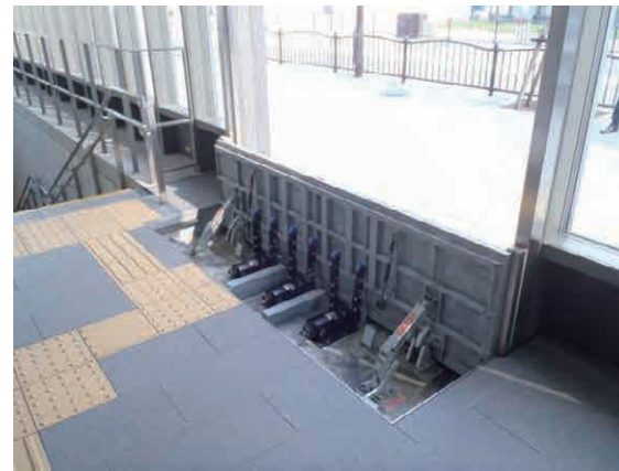
Figure 3.4.35 Example of water sealing plates
