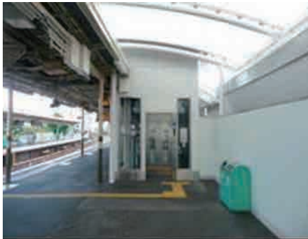
Source: JICA Study Team Figure 3.4.33 Elevator
