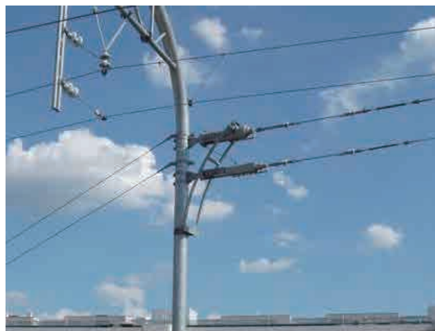
Figure 3.6.9 Image of automatic tensioner
