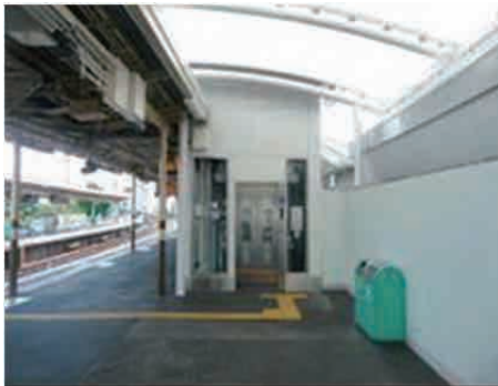
Source: JICA Study Team Figure 3.4.33 Elevator
