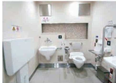
Source: JICA Study Team Figure 3.4.34 Multifunctional toilet
