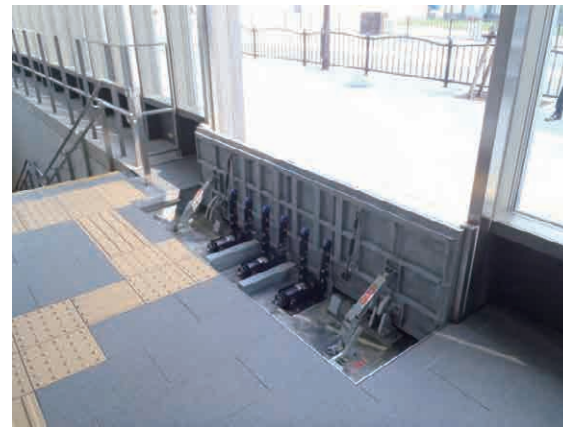
Figure 3.4.35 Example of water sealing plates
