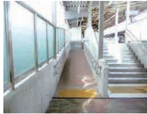
Source: JICA Study Team Figure 3.4.30 Handrail
