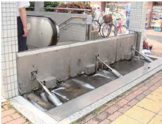
Figure 3.4.35 Example of water sealing plates
