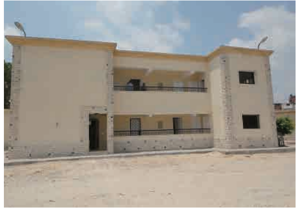
No.13 District Office
