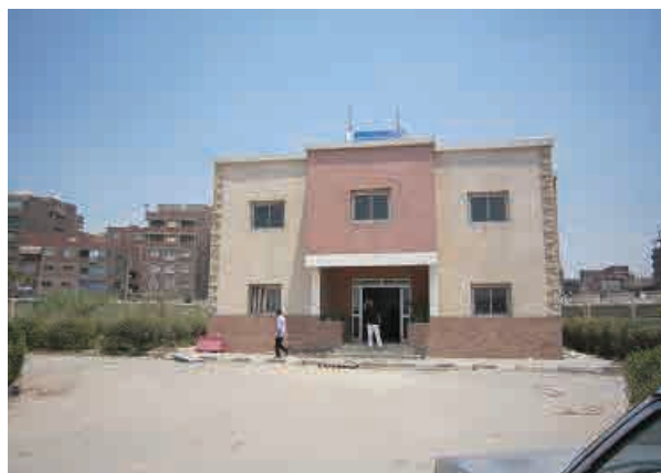
Central District Office (Ring Road)
