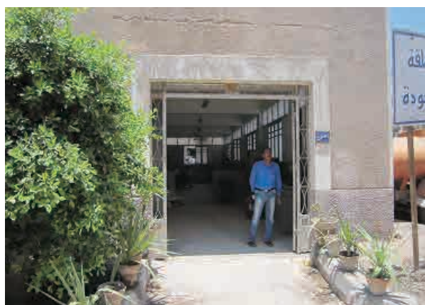
品質管理試験室 (East Delta District Office)
