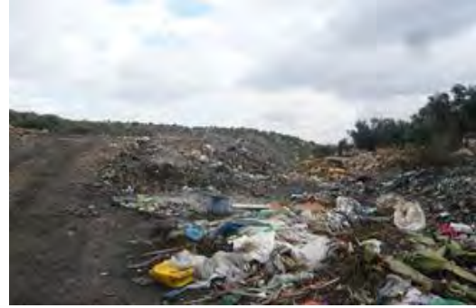
Pic-10 Existing Open Dump Site in Salfit JC (1): Household waste is dumped without cover soil.
