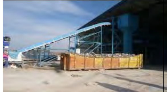
Pic-2 Landfill in Jenin JC (2): Recyclable material is selected by hand sorting from the belt conveyor system.
