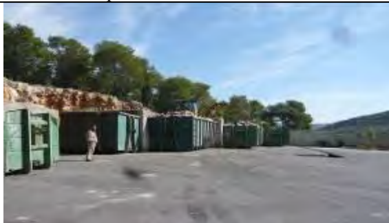
Pic-5 Waste Transfer Station in Tulkarem JC (1): Household waste is compacted by compaction unit at the waste transfer station, transferred/disposed at the Jenin landfill.
