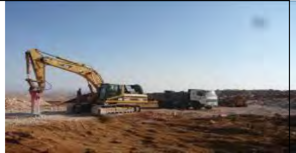
Pic-4 Sanitary Landfill in Hebron JC: The sanitary landfill is under construction by the World Bank Assistance.
