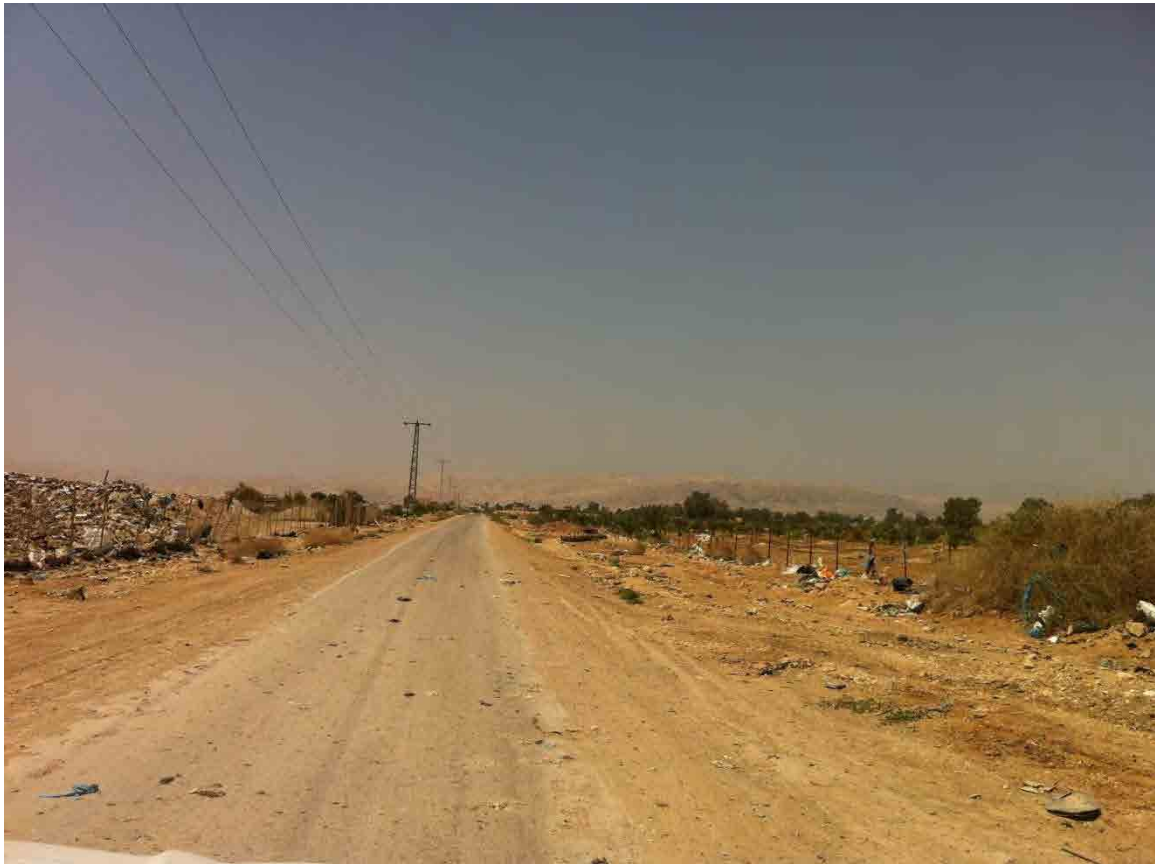
Plate 3.20: The road leading to the landfill and the expansion site
