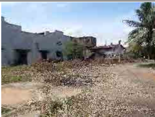
Photo-5 Condition of Proposed New Water Treatment Plant Site for Battambang
