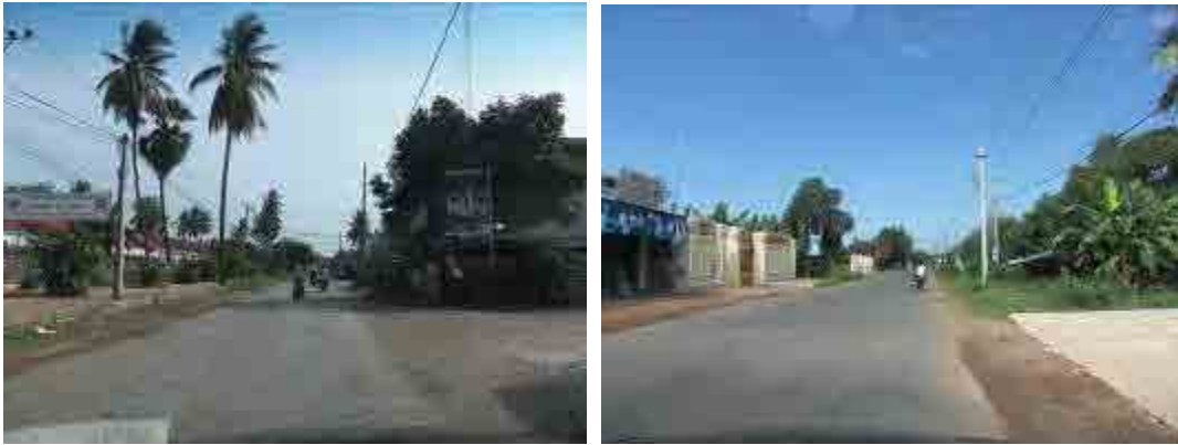
Photo 2.2.2.6-1 Current state of installation location of pipeline
