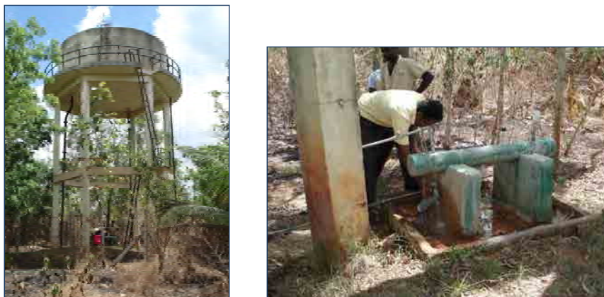
Figure 2.25 CBO Water Tank (left) and Sampling Drain (Right)
