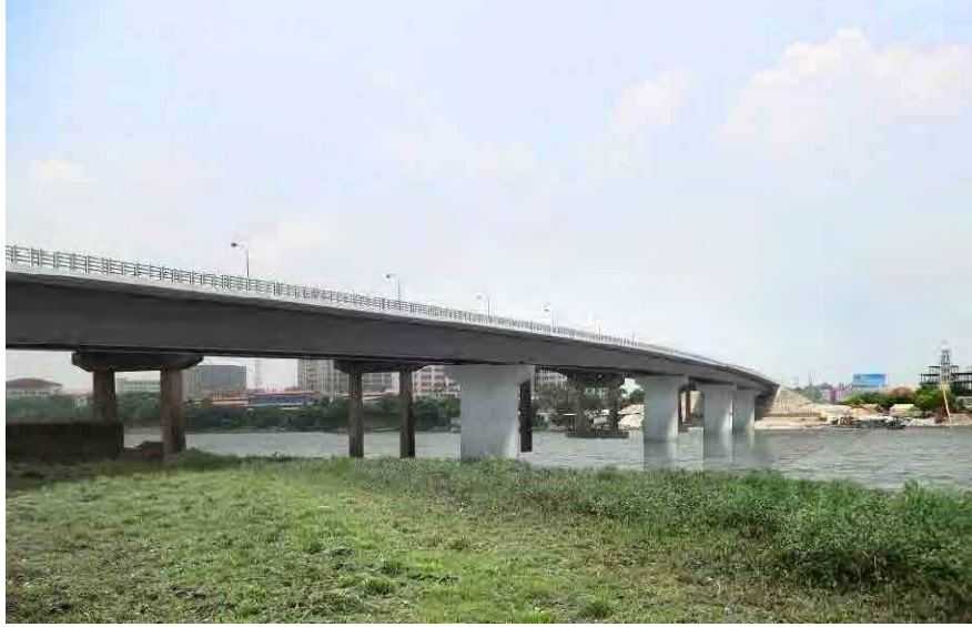
Figure 7.9 New bridge (imaged) and Existing Bridge (background) at Kanchpur Bridge Site
