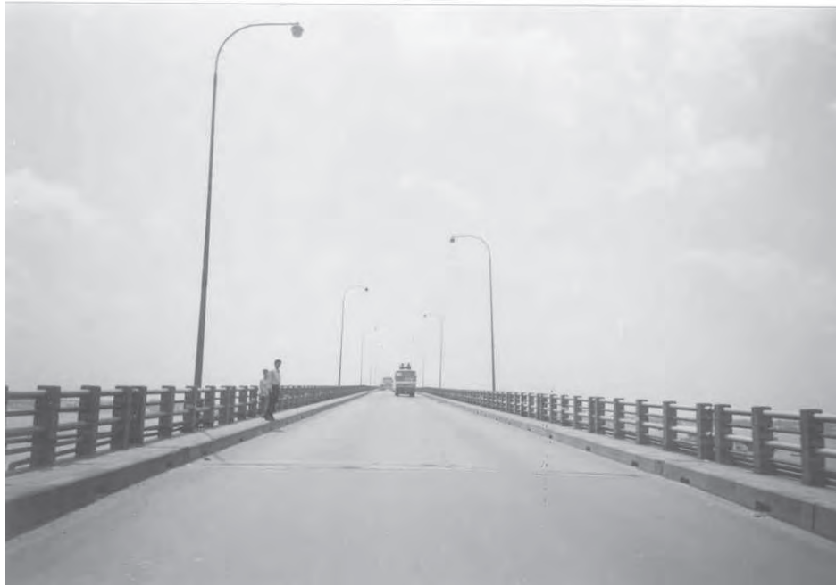
TOP VIEW OF BRIDGE
