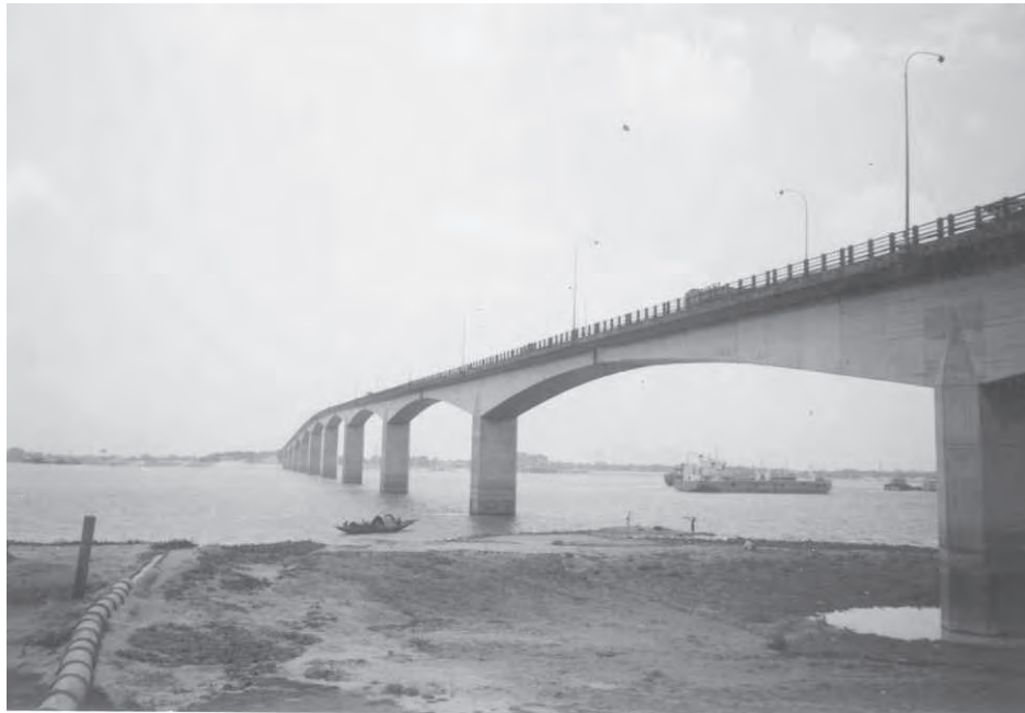
SIDE VIEW OF BRIDGE
