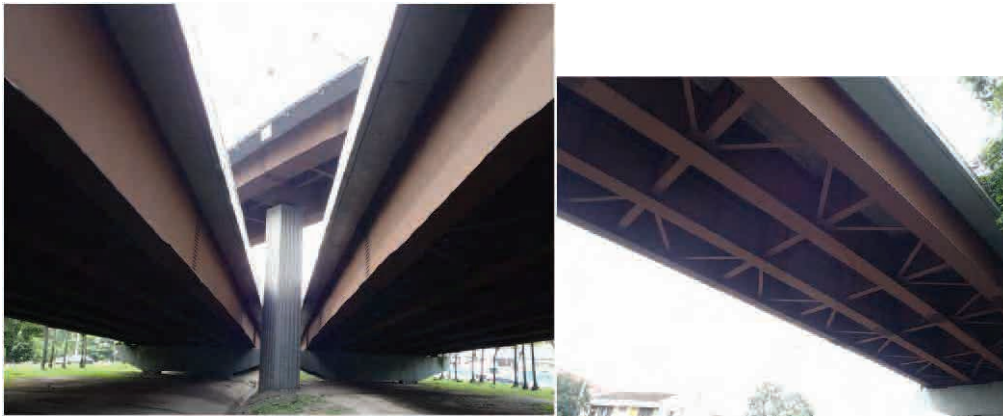
(a) Kepong Interchange (Malaysia)
