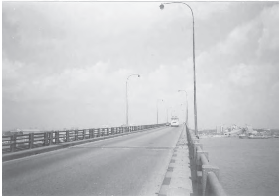
ANOTHER TOP VIEW OF THE BRIDGE
