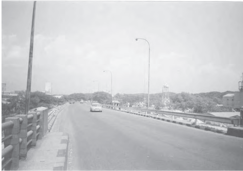
APPROACH ROAD BRIDGE
