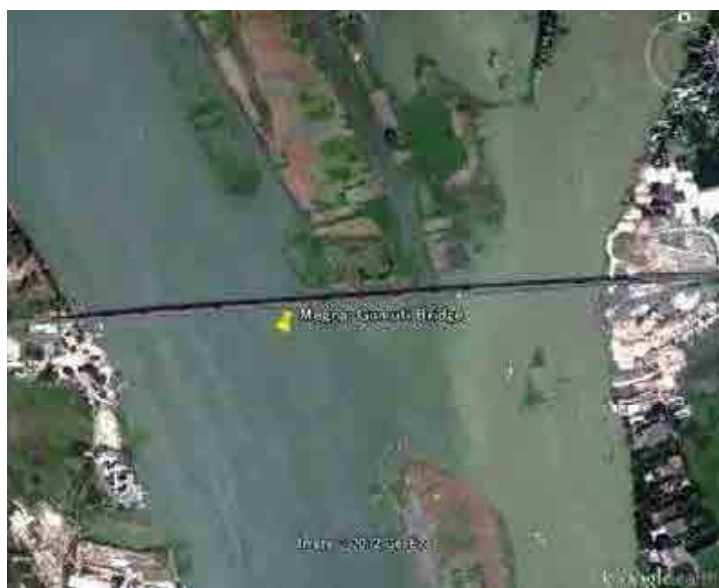
Figure 4.24 Chars (sand bar island) at Gumti Bridge Site
