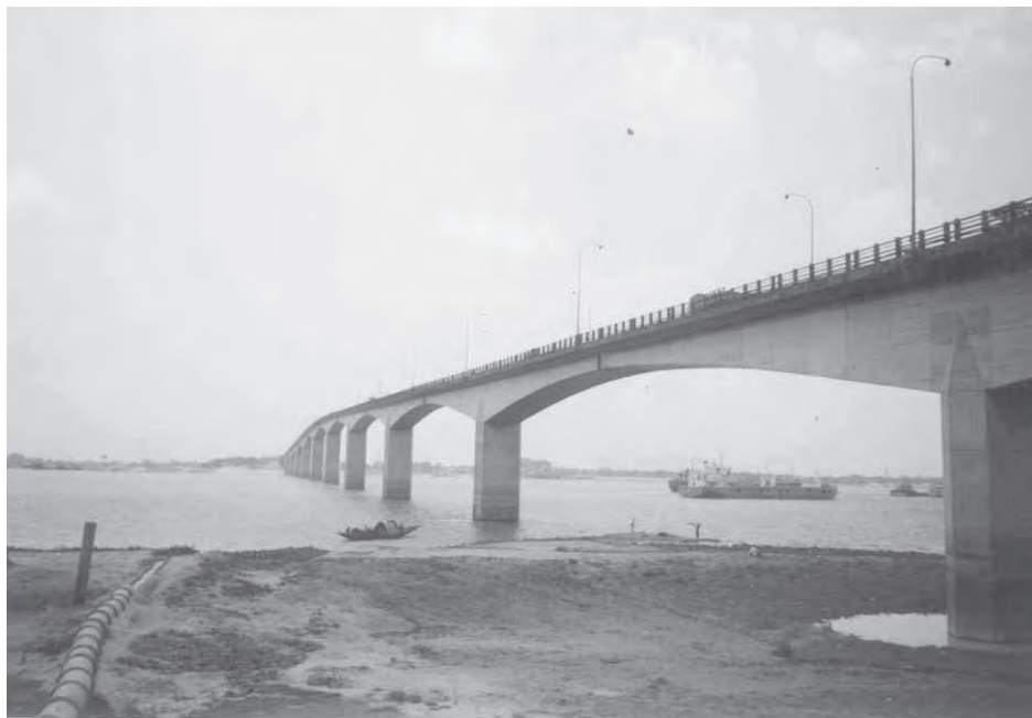
SIDE VIEW OF BRIDGE
