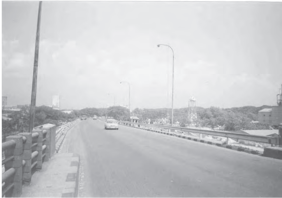
APPROACH ROAD BRIDGE
