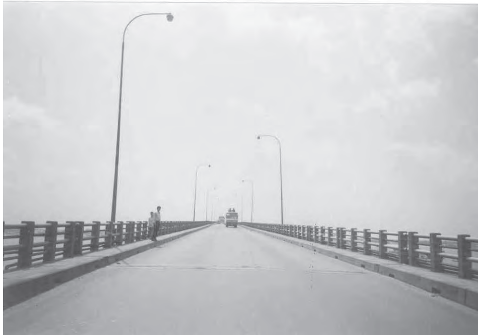
TOP VIEW OF BRIDGE
