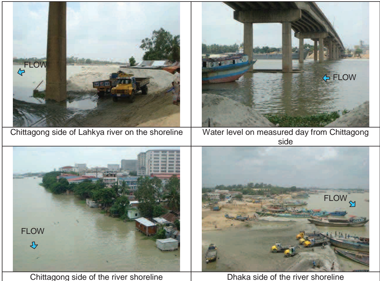
Figure 1.4.13 Water Level on the Measured Day at Kanchpur Bridge (July 30th 2012)
