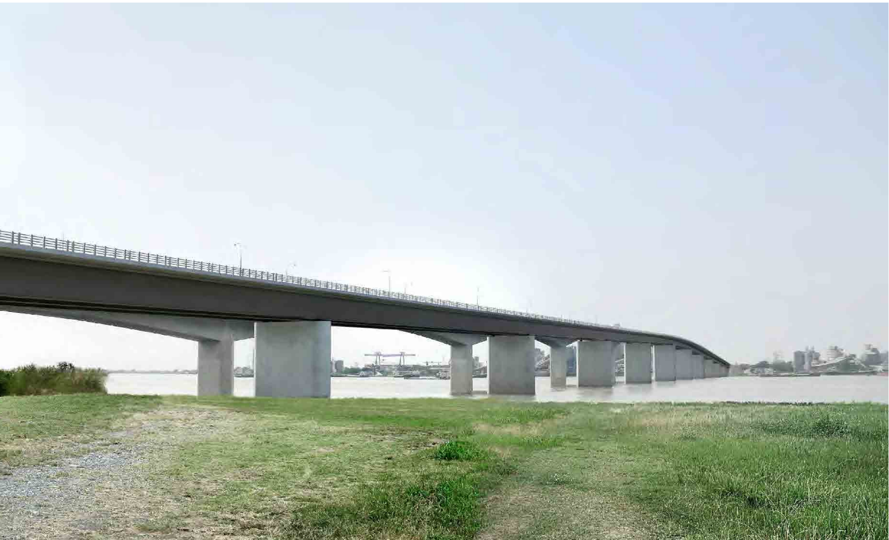
Figure 9.2.6 CG of Completed the 2 nd Meghna Bridge (Chittagong side)
