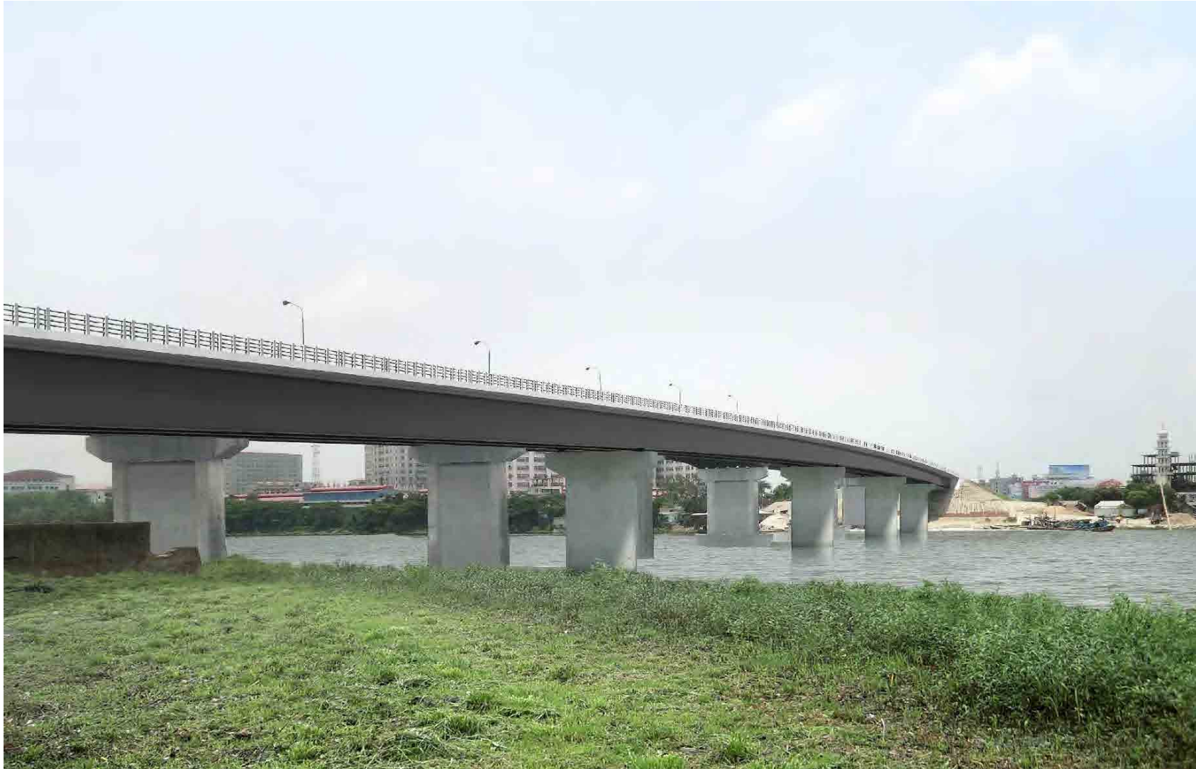
Figure 9.2.3 CG of Completed the 2 nd Kanchpur Bridge (Dhaka side)
