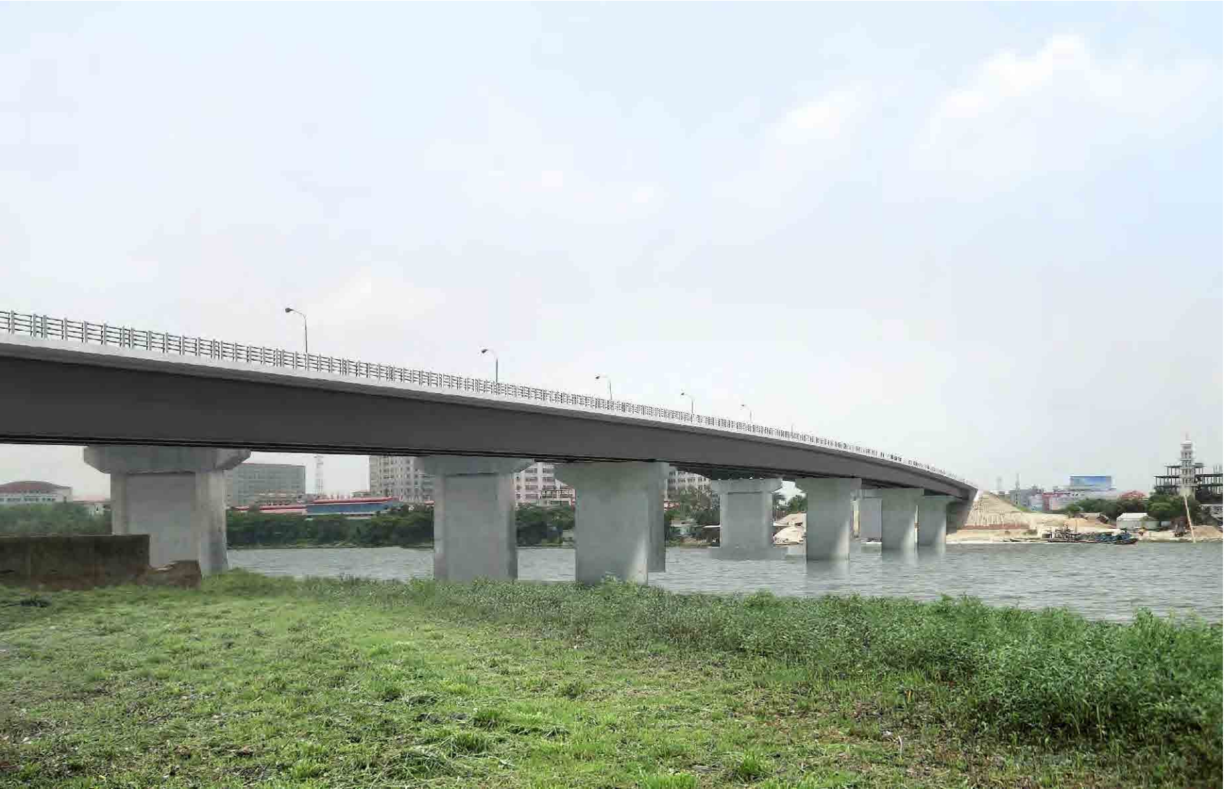
Computer Graphics of completed 2 nd Kanchpur Bridge (Dhaka side)
