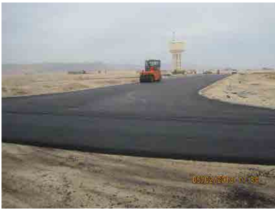
Internal Road Pavement
