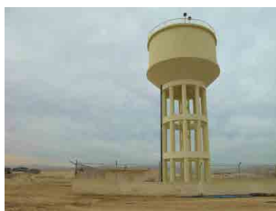
Elevated Water Tank
