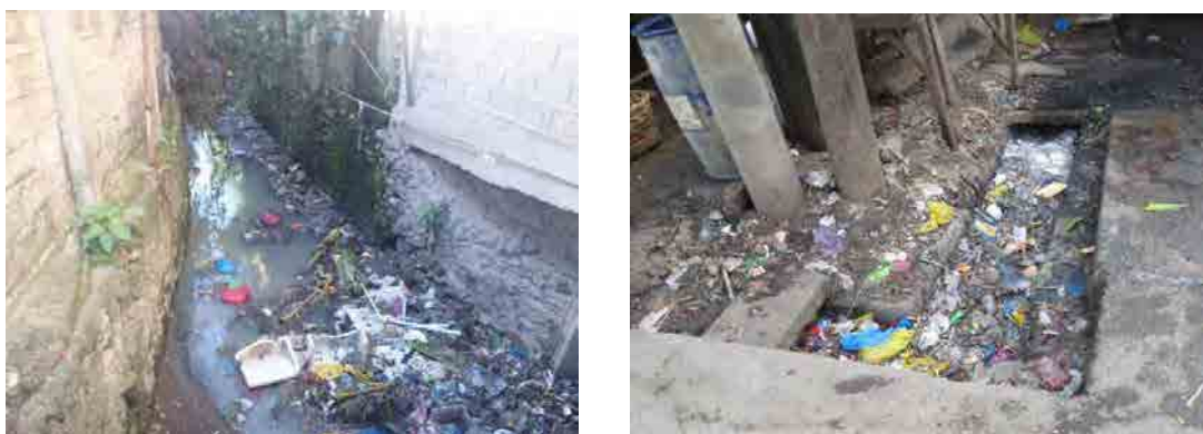
Figure 6-10 Condition of Existing Drainage Facility
