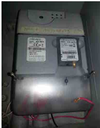
Figure 6-34 Sample of Advanced Meters at VECO
