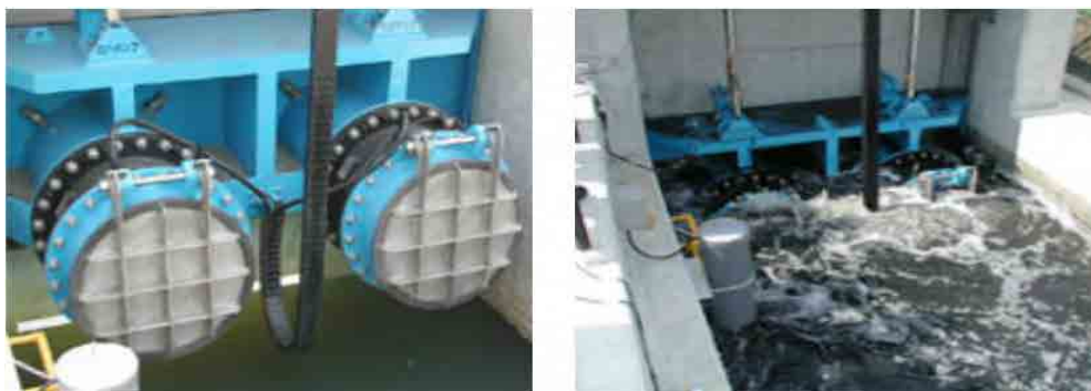
Figure 6-19 Sample of the Pump with Gate
