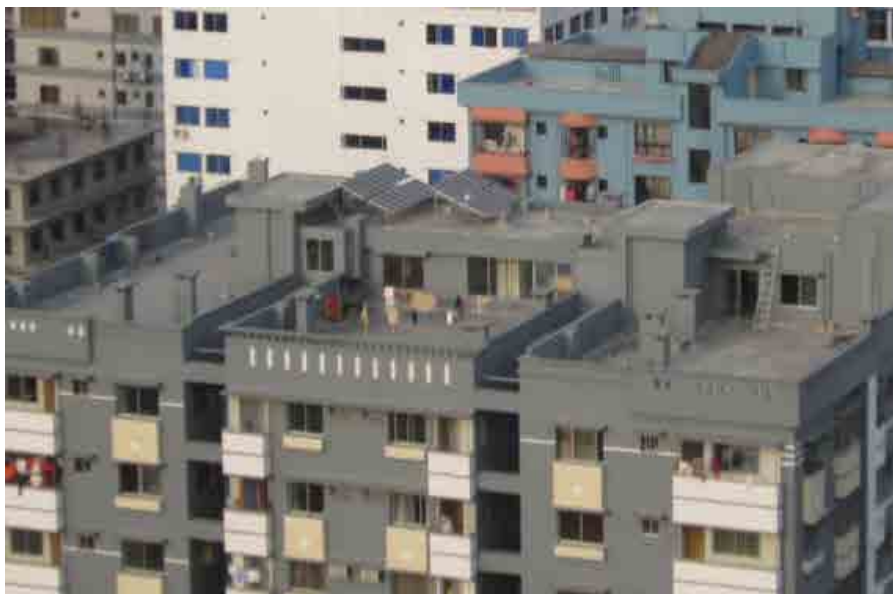
Figure 2.4-3 PV Panels Installed on the Building Roof
