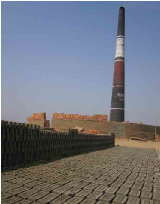
(a) FCK facility Source: Survey Team
