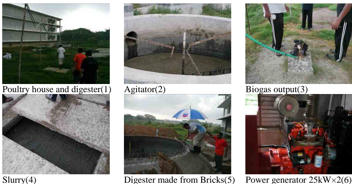
Figure 2.3-13 50kW Poultry Waste Biodigester Plant
