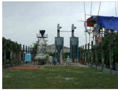
Whole view of the plant
