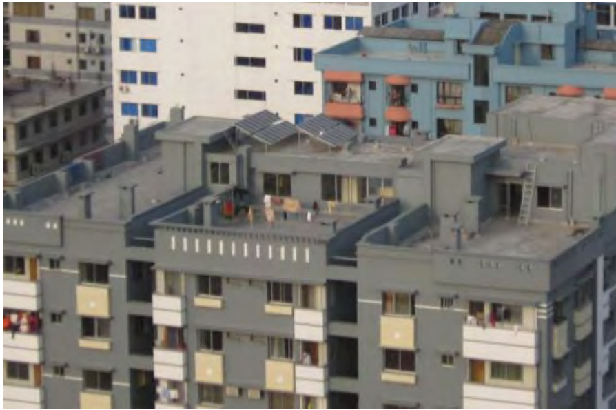
Figure 2.4-3 PV Panels Installed on the Building Roof
