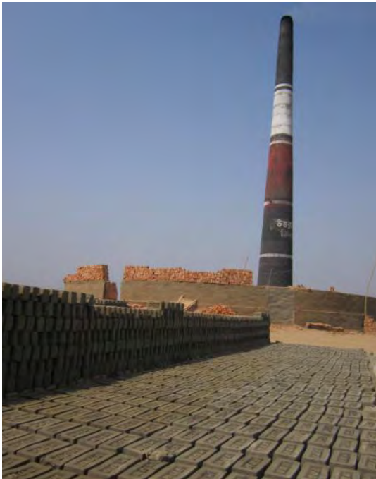
(a) FCK facility Source: Survey Team
