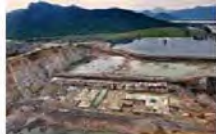
Poivaram cofferdam designs yet to be finalise... thehindu.com
