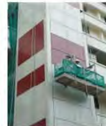
Suspended Scaffold for... kimsingscaffolding.com
