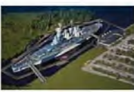
SECU Memorial Walkway and cofferdam... west.com
