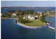
Temporary Cofferdams, Flood Protectio... portadam.com
