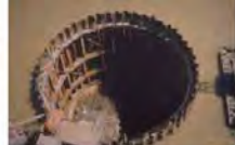
Cofferdam | SpringerLink link.springer.com
