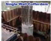
2) Single wall cofferdam, (http://s... researchgate.net
