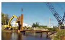
Building A Cofferdam Start To Finish - YouTub... youtube.com
