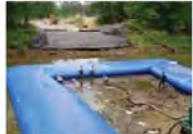
The Top 6 Uses For a Cofferdam | Hydr... hydrologicasolutions.com
