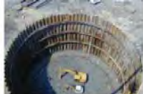
Cellular Cofferdams Vital to Marine Constru... planetlock.com
