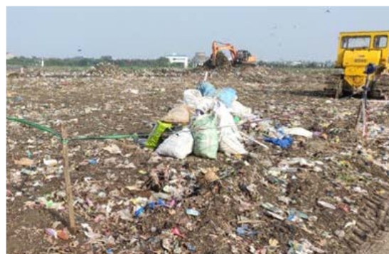
Photo 7 Soil covering work (as of December 2019)
