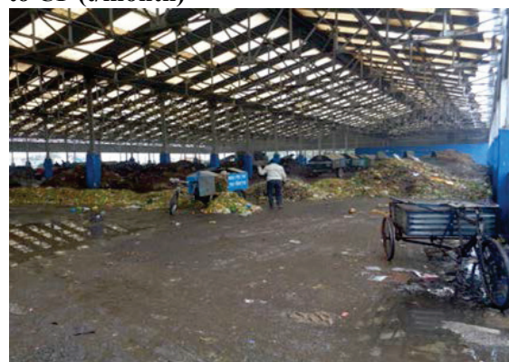
Photo 1 Situation in CP in Uttarpara-Kotrung (as of December 2019)
