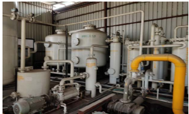
Co 2 , H 2 S gas removal and extraction of CH 4
