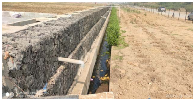
Gabion boxes with bolder provided along the periphery of site
