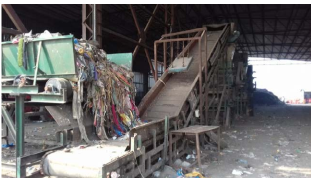
120mm screen machine in processing plant
