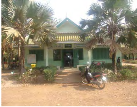
Elevation : Façade (Administration)
