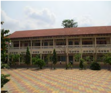
Elevation : Façade Occupied by local residents
