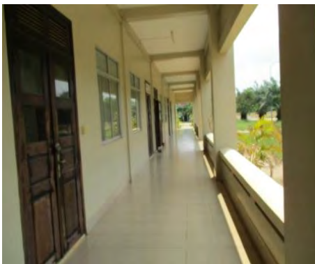
Corridor of front side at 1st.FL.
