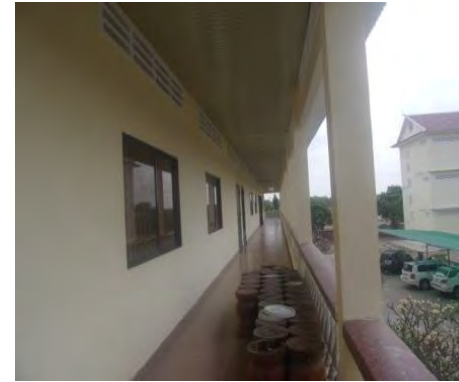
Corridor at 1st. FL.
