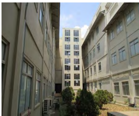
Patio of Class room Building
