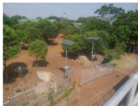
Surrounding of facility
