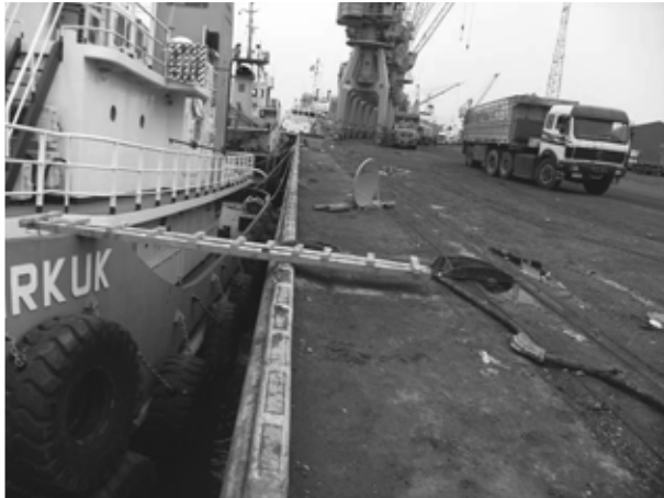
Photo 3.3.18 Berth Nos. 16 and 17
