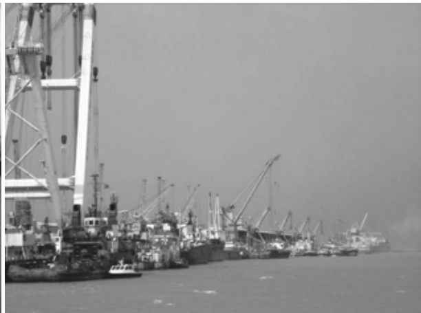
Photo 3.3.45 Overview of Berth Nos. 2 to 6
