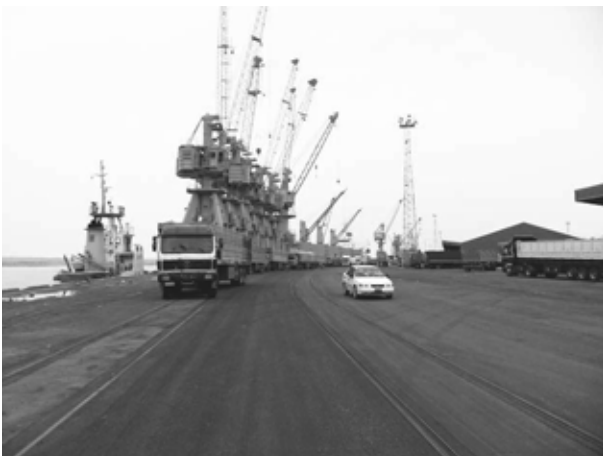
Photo 3.3.16 Q/C (at Berth No. 20)
