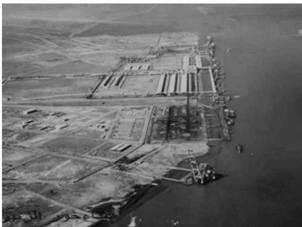
Photo 3.3.22 Aerial View of KZP
