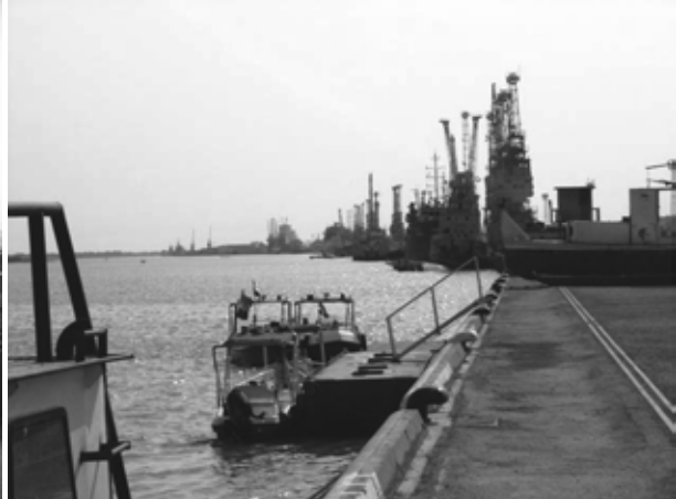
Photo 3.3.53 Overview from Upstream
