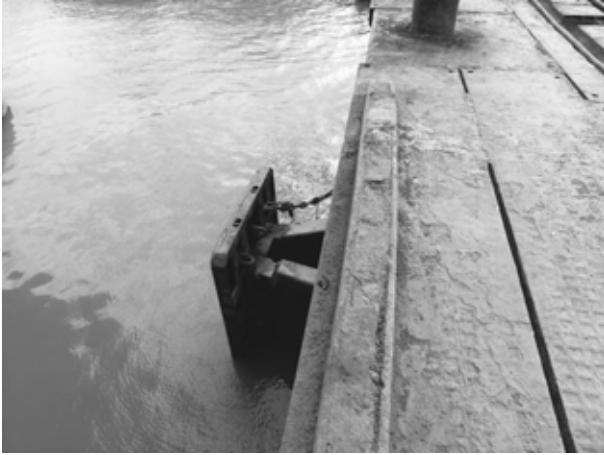
Photo 3.3.42 Fender (at Berth Nos. 2 to 4)
