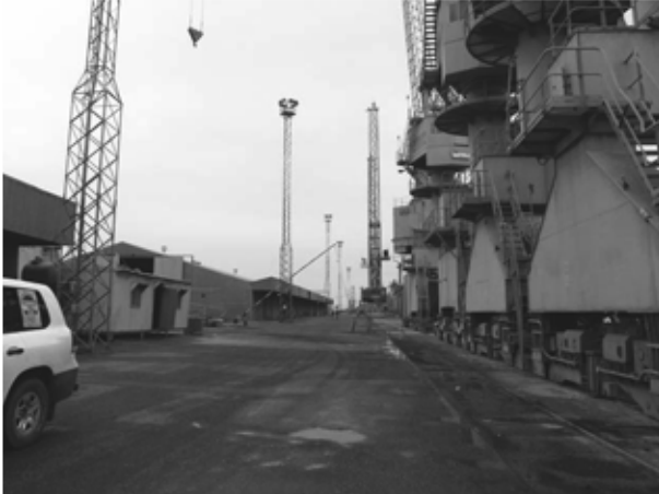
Photo 3.3.6 Non-operational Q/C (at Berth No. 7)
