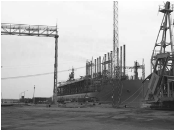
Photo 3.3.2 Power Barge (at Berth No. 9)
