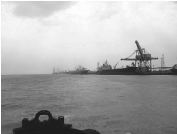
Photo 3.3.44 Overview of Berth Nos. 9 to 6
