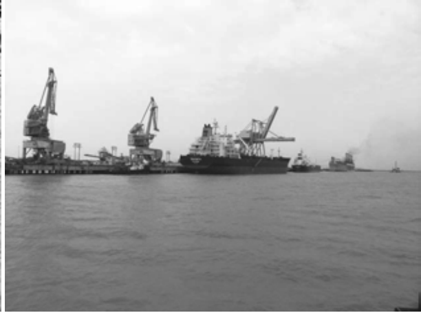
Photo 3.3.43 Overview of Berth Nos. 9 to 11
