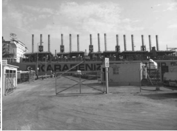
Photo 3.3.25 Power Barge (at Berth No. 11)
