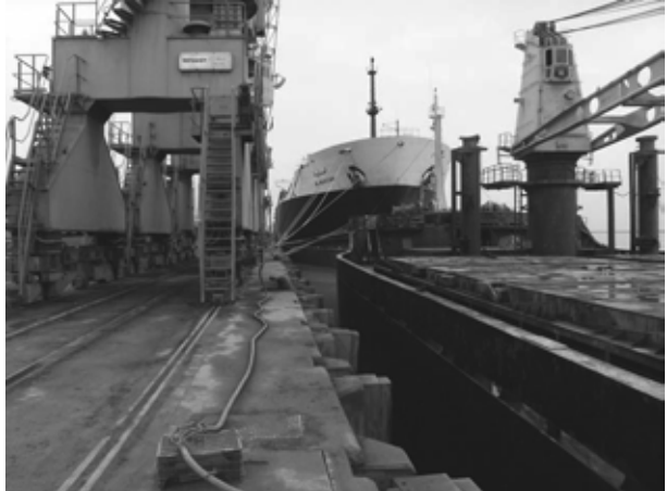
Photo 3.3.7 Q/C and Fender (at Berth No. 7)
