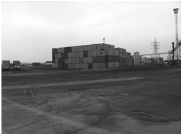
Photo 3.3.3 Container Yard (at Berth No. 8)
