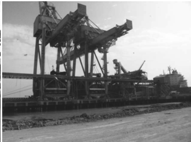
Photo 3.3.27 Detached Pier Type Berth (at Berth Nos. 6 to 8)
