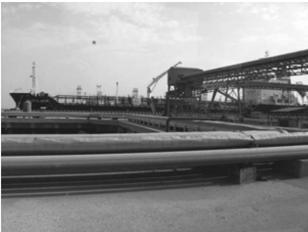
Photo 3.3.26 Oil Tanker (at Berth Nos. 9 and 10)
