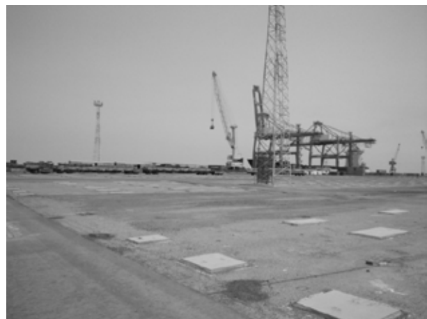
Photo 3.3.21 Container Cargo Yard (at Berth No. 21)
