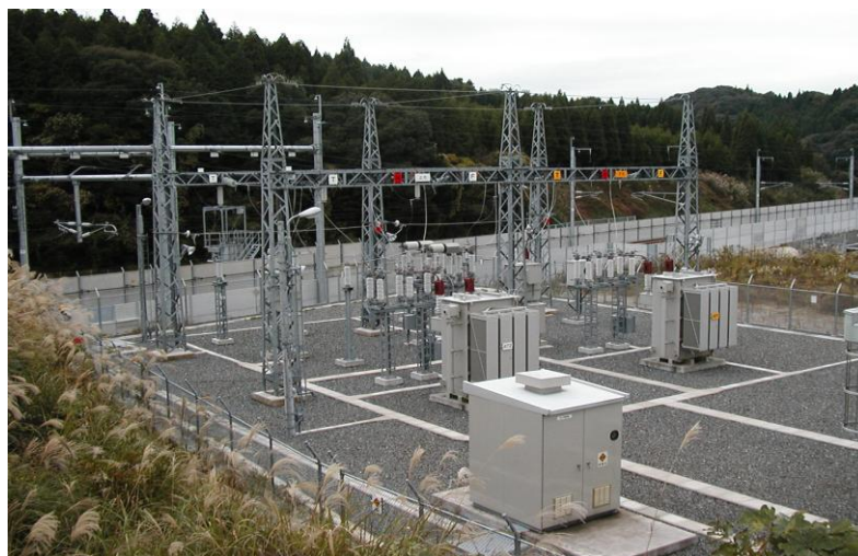
Figure 5.3.101 A sample Auto-Transformer Post (ATP) in Japan
