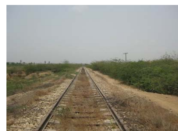
③ Depot Hill yard
