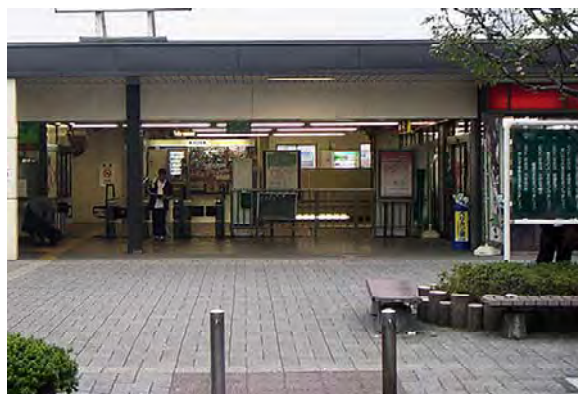
Entrance on ground level
