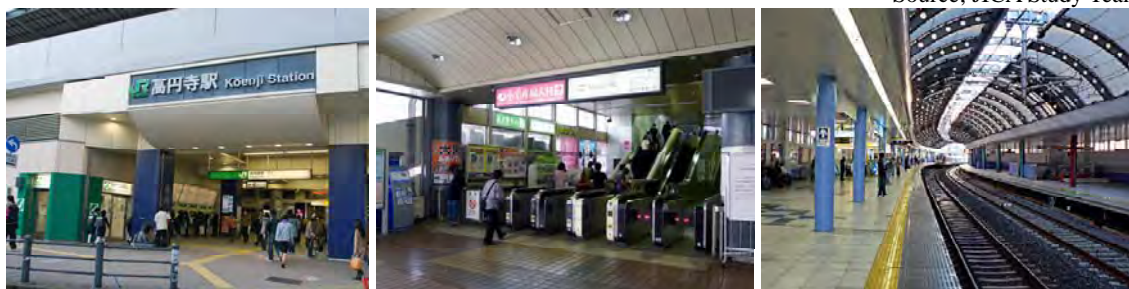
Entrance of Viaduct Station
