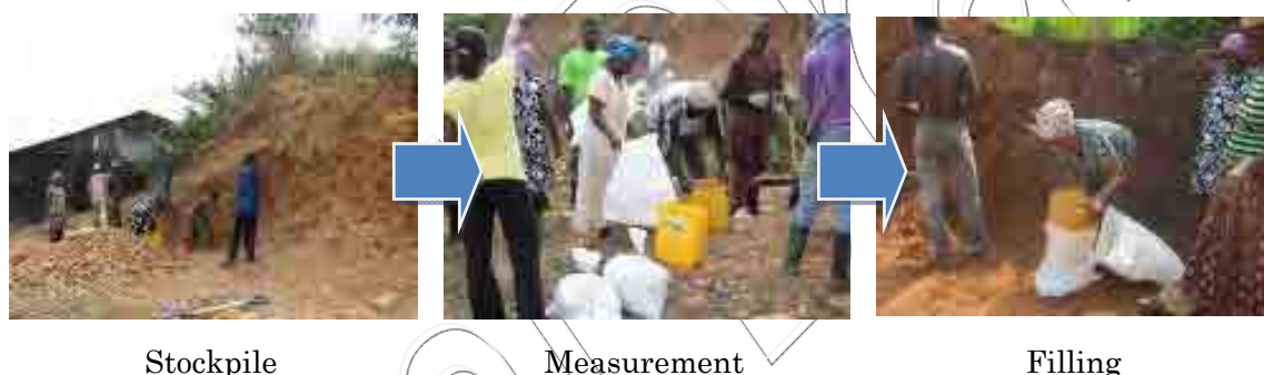
Figure 5-6 Procedure from Stockpile to Filling Do-Nou
