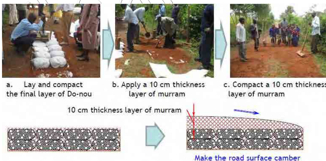
Figure 5-11 Covering and Compaction
