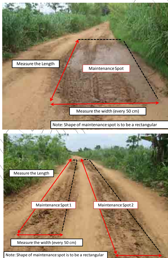
Figure 4-1 Identification of Maintenance Spot and Size
