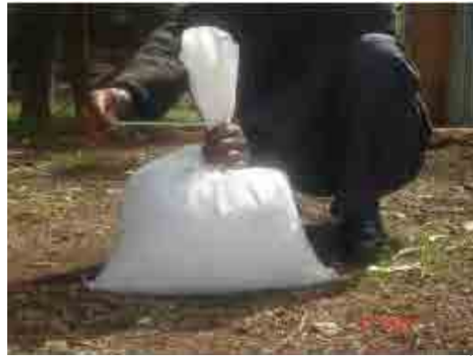
Figure 5-7 Position to be Tied for Standard Do-Nou
