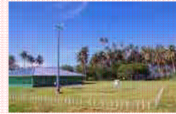
Equipment installed at Samoa meteorology headquarters
